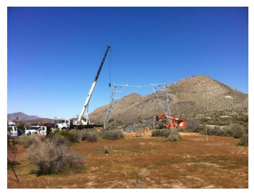
Figure 1: Conventional structure assembly at EP 243, Link 1.
