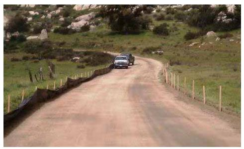
**Figure 9:** Silt/wildlife exclusionary fence installation along access road to Kreutzkamp Construction Yard, Link 2.
