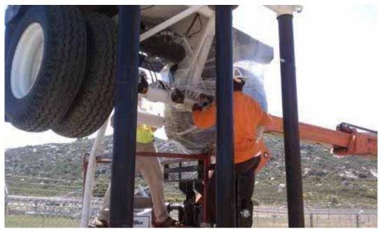
**Figure 7:** Crews attempting to deter nesting birds with plastic wrap on equipment at Kreutzcamp Construction Yard, Link 2.
