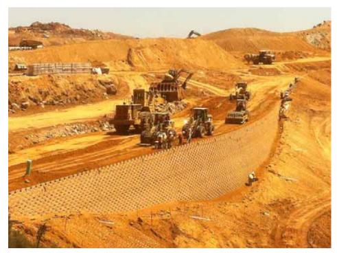
**Figure 6:** Block retaining wall along northern drainage, Link 3.
