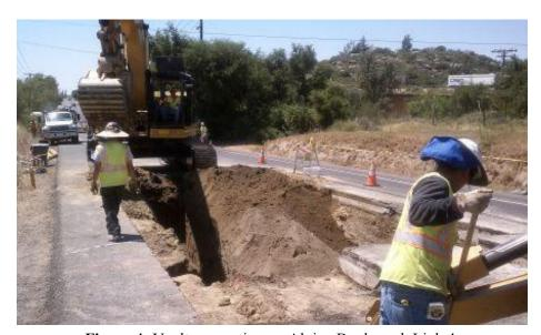
Figure 4: Vault excavation on Alpine Boulevard, Link 4.
