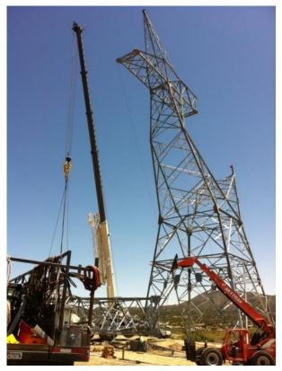
**Figure 1:** Conventional tower assembly at EP210, Link 1.
