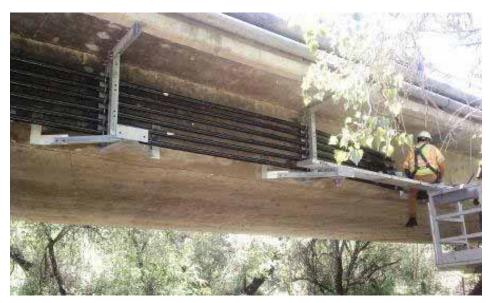
Figure 3: Attachments of conduit to Viejas Bridge, Link 4.
