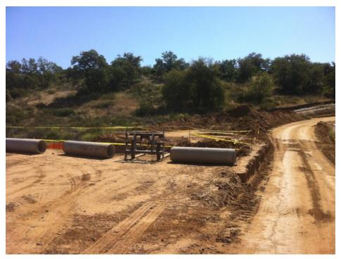
**Figure 8:** Culvert installation near Smith property, Suncrest Substation, Link 3.
