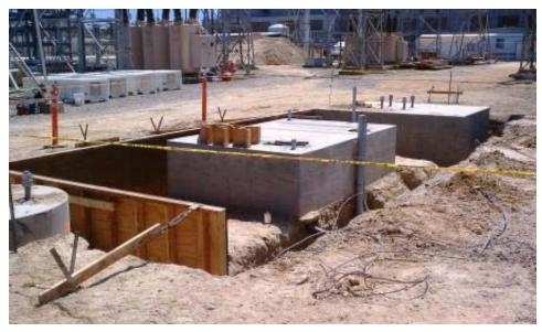
Figure 7: Wood work for pouring concrete foundation at Encina Substation.
