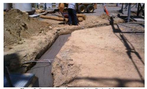
Figure 8: Concrete poured over conduit at Encina Substation.
