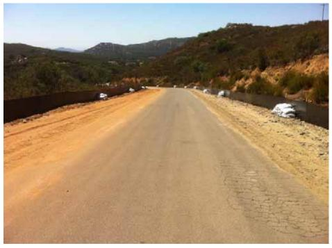
**Figure 5:** Road improvements on Bell Bluff truck trail to allow for transformer delivery to Suncrest Substation. (Link 3)
