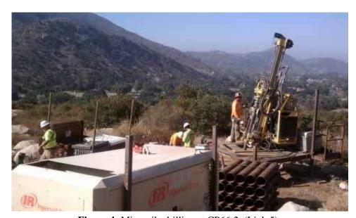
**Figure 4:** Micropile drilling at CP66-2. (Link 5)
