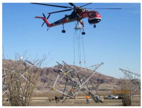
Figure 9: Air crane tower pick at S-2 Construction Yard. (Link 1)
