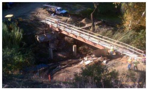
**Figure 5:** Bridge removed at Bauer Property. Pedestrian footbridge in place. (Link 4)
