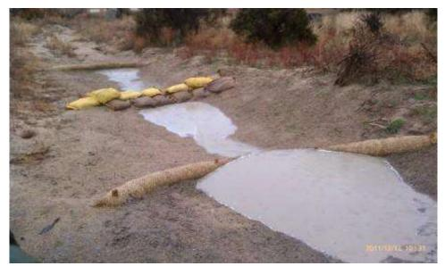
Figure 7: Check dams along La Posta Road in USFS. (Link 2)
