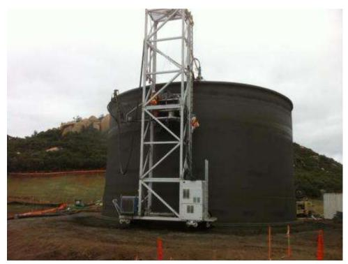
Figure 10: Shotcrete application on water tank near trailers. (Link 3)
