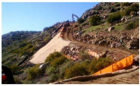
Figure 5: Grading and boulder removal on access road to CP49-1 pull site. (Link 5)
