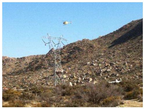
Figure 2: Flying sock line from EP255-2 pull site to EP269-1 pull site. (Link 1)
