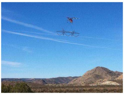
**Figure 3:** Aircrane flying bridge to EP253-3. (Link 1)
