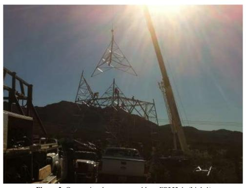
**Figure 2**: Conventional tower assembly at EP252-1. (Link 1)
