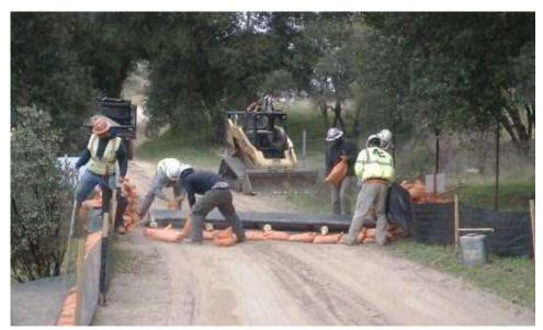
**Figure 4:** Crews assembling a cattle guard and arroyo toad exclusion device on access road to EP78. (Link 2)
