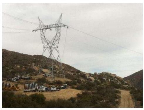
Figure 2: Pulling wire between EP219-1 and EP220-1. (Link 1)
