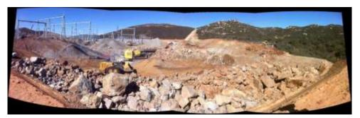
Figure 10: Rock being crushed for Class 2 base and select fill. (Link 3)
