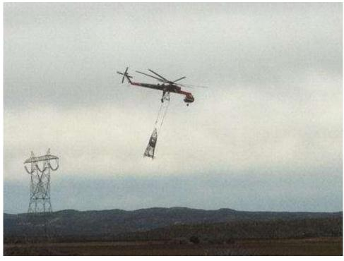
**Figure 12:** Air crane flying tower structures out of JVR Yard. (Link 1)
