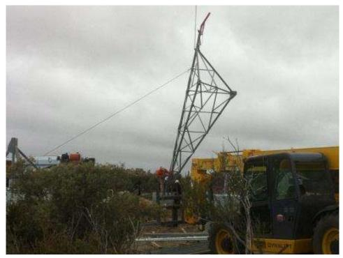
**Figure 1:** Conventional tower assembly at EP191. (Link 1)
