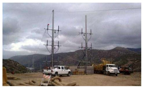
**Figure 2:** Wire pulling operations at CP88-1. (Link 5)
