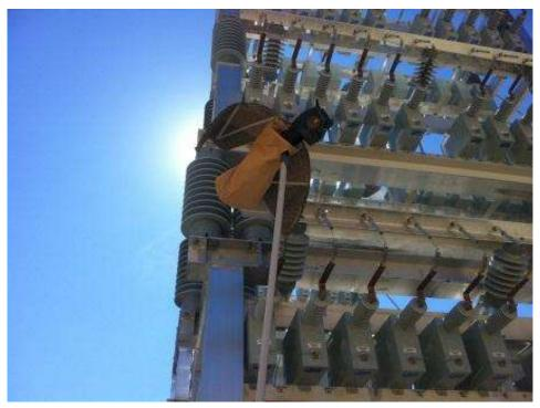
Figure 7: One of various types of bird deterrents at Suncrest Substation. (Link 3)
