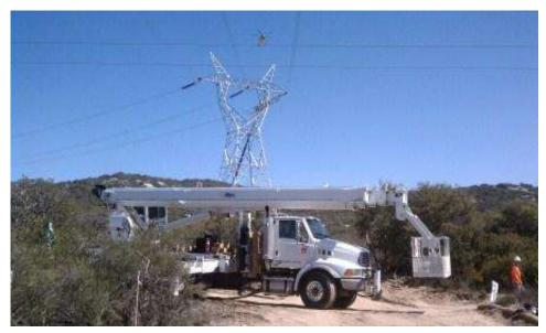
**Figure 3:** Fiber being flown at Tower EP91. (Link 2)
