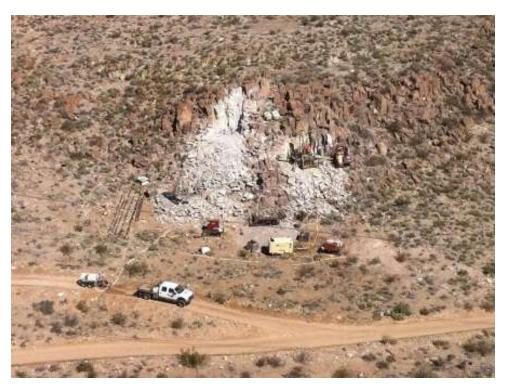
**Figure 1:** Micropile drilling at Tower EP245-3. (Link 1)
