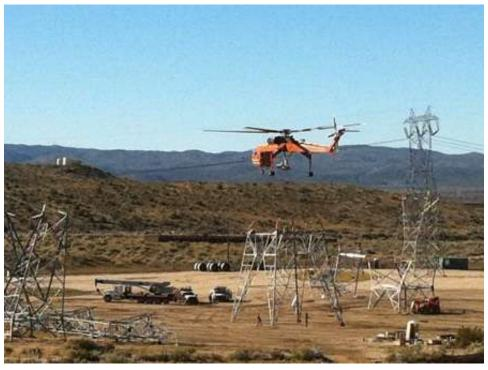
**Figure 3:** Aircrane "picking" a pre-assembled tower piece for Tower EP228. (Link 1)
