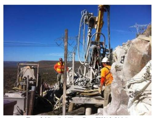
**Figure 2:** Micropile drilling at Tower EP254-3. (Link 1)
