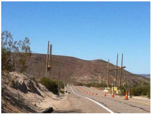
Figure 3: Guard structures at EP251/EP252 over Old Highway 80. (Link 1)
