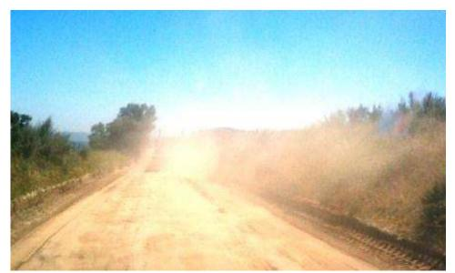
Figure 9: Dust from project vehicle on access road to Bartlett Hauser Construction Yard. (Link 2)
