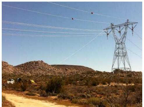
Figure 1: OPGW pulling at Tower EP244. (Link 1)
