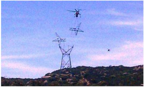
**Figure 4:** Air crane delivering pre-assembled tower piece at Tower EP83. (Link 2)
