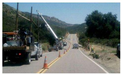
**Figure 3:** Guard structure installation on Lyons Valley Road near Tower EP24. (Link 2)
