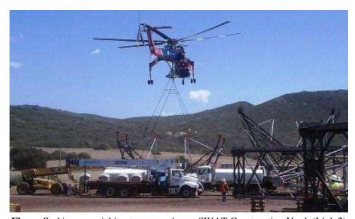
Figure 8: Air crane picking tower section at SWAT Construction Yard. (Link 2)
