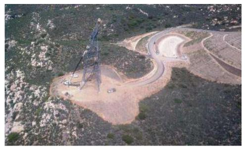
**Figure 5:** Wire pulling activities at Tower EP1, adjacent to Suncrest Substation. (Link 2)
