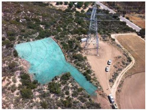
**Figure 2:** Hydromulching at EP89-1 pull sites. (Link 2)
