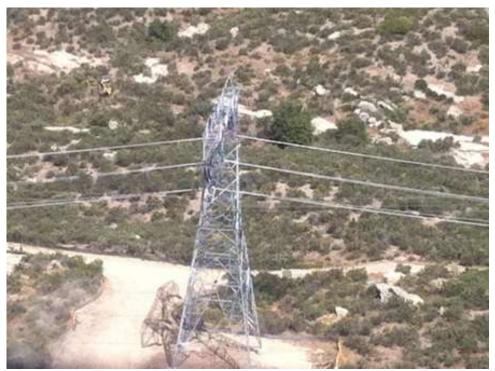
Figure 1: Flying OPGW fiber at EP68. (Link 2)
