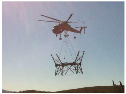
**Figure 5:** Air crane flying a tower section from Bartlett Hauser Yard. (Link 2)
