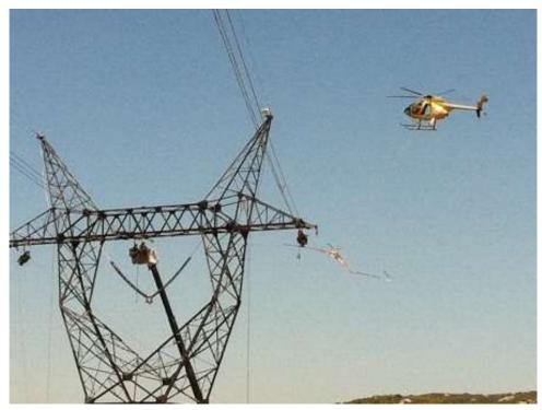
Figure 3: Flying sock line at EP12-3. (Link 2)
