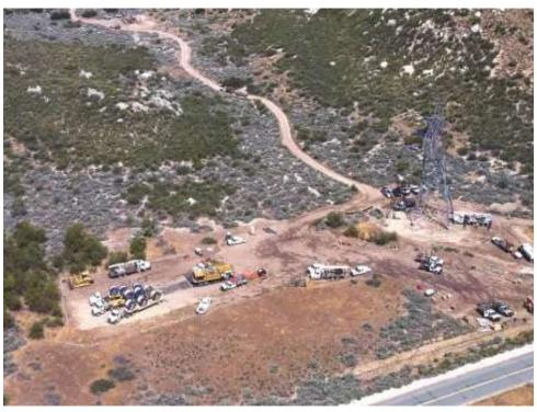
**Figure 4:** Aerial view of pulling operations at EP113-5 pull site. (Link 2)
