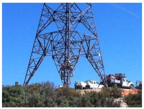
**Figure 1:** Installing anti-climbing guards at EP126-1. (Link 2)
