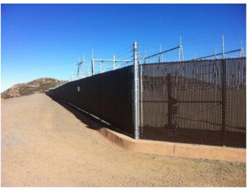
**Figure 2:** Fence slats installed along the southern side at Suncrest Substation. (Link 3)
