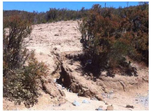
Figure 6: Failed BMP at EP124/EP125 pull site. (Link 2)
