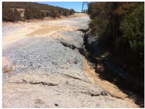
**Figure 7:** Gulley created by significant rain event along La Posta Truck Trail near EP124/EP125 pull site. (Link 2)
