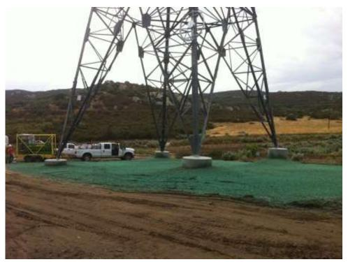
Figure 4: Hydromulching at Tower EP113-5. (Link 2)
