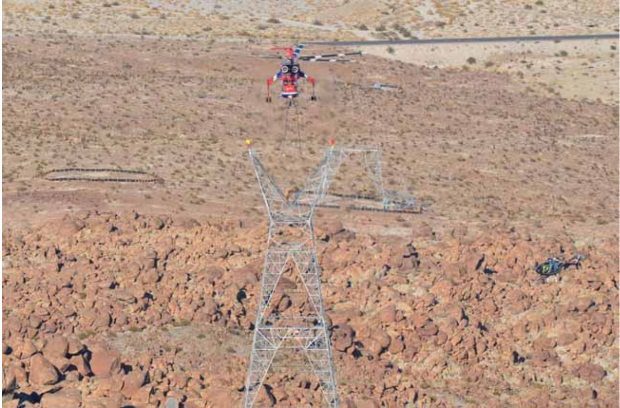
Setting of the layback at EP279-1. Photo courtesy of Rebecca Carson.
