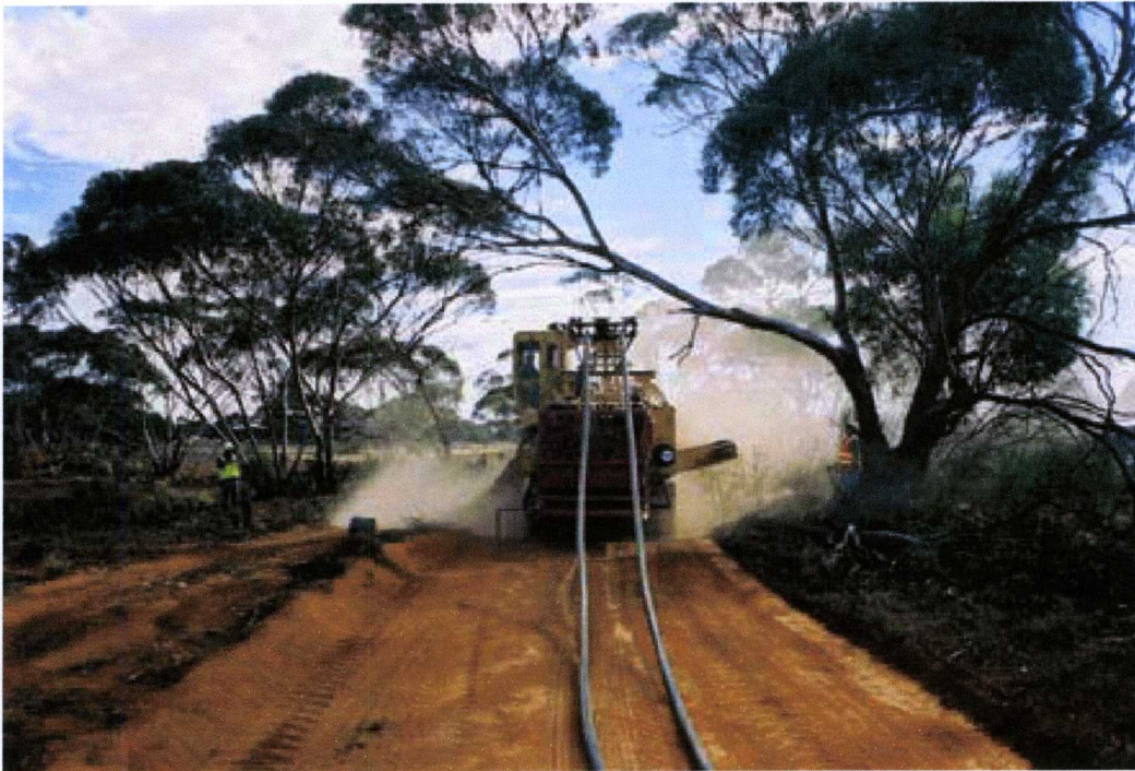
Cable laying for MurrayLink project
