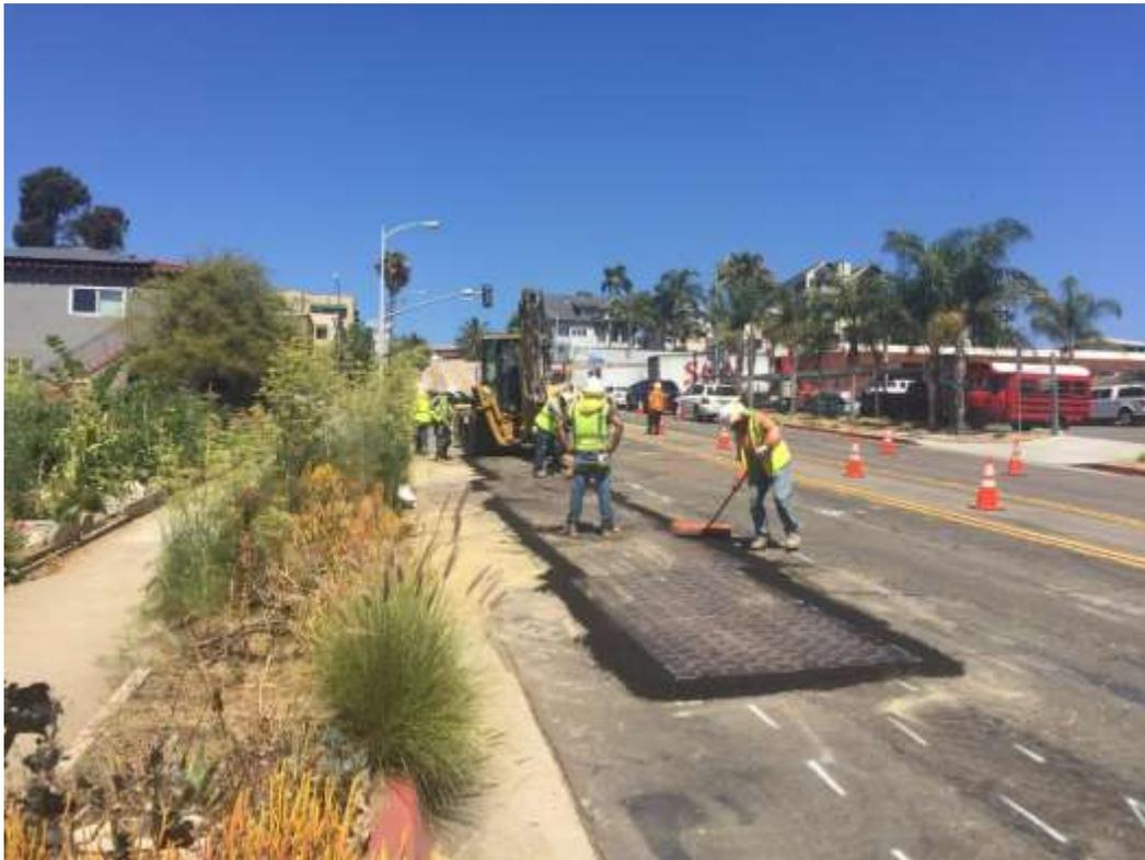
Figure 3 – Trench backfilling and clean-up activities along W. Laurel Street, 12-kV Underground.
