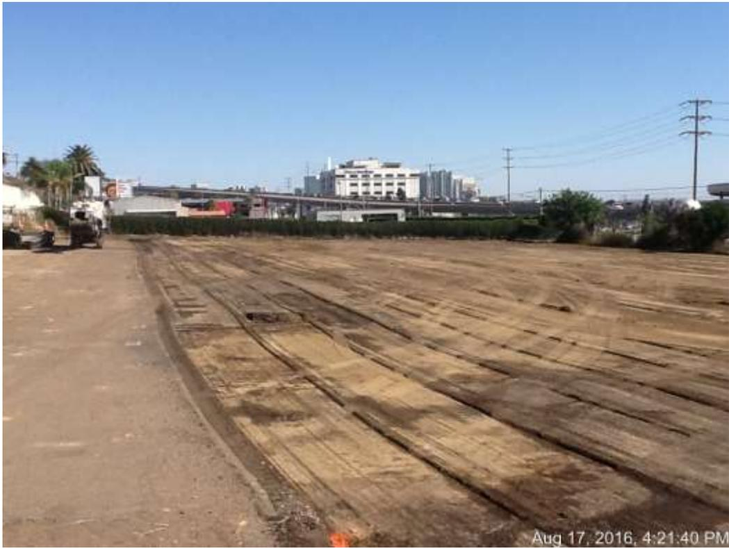
Figure 1 – Asphalt removal at the Vine Substation site. Asphalt was hauled off site as it was removed.
