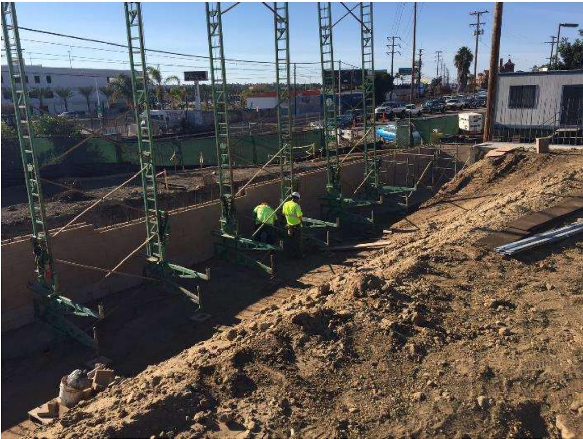
Figure 3 – Scaffolding to complete the higher portions of the block wall along the southwestern site boundary.
