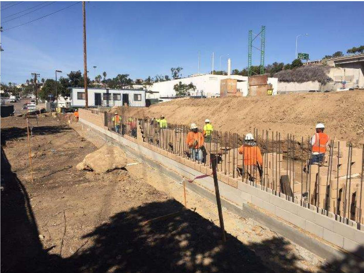
Figure 2 – Block wall installation along the southwestern site boundary.
