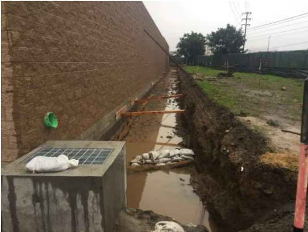
Figure 3 – Location of the storm water accumulation adjacent to the block wall footing (during the storm event).
