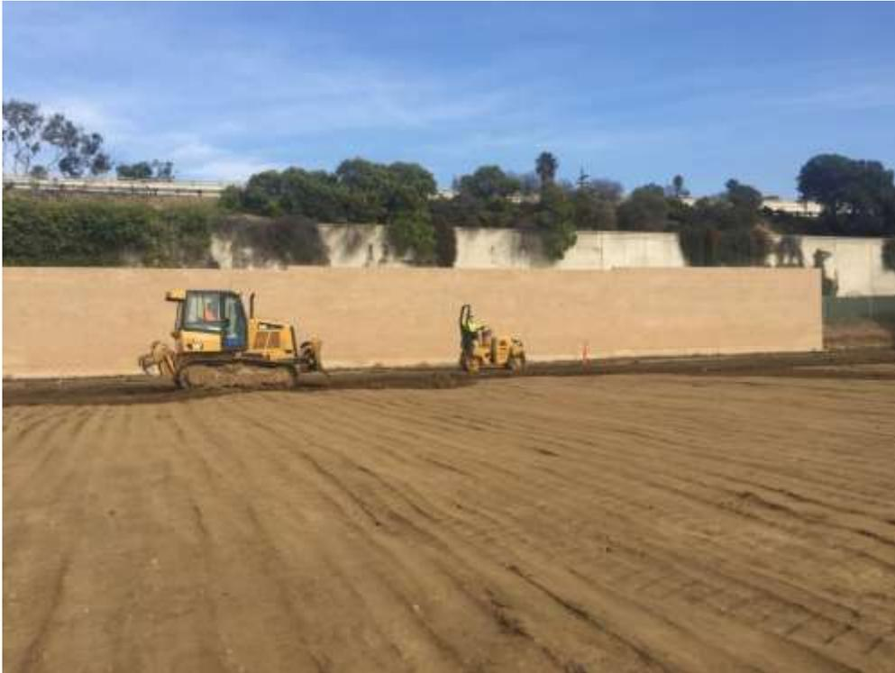
Figure 1 – Construction contractor preparing the ground surface prior to the rain event in order to minimize accumulation of storm water on the site.
