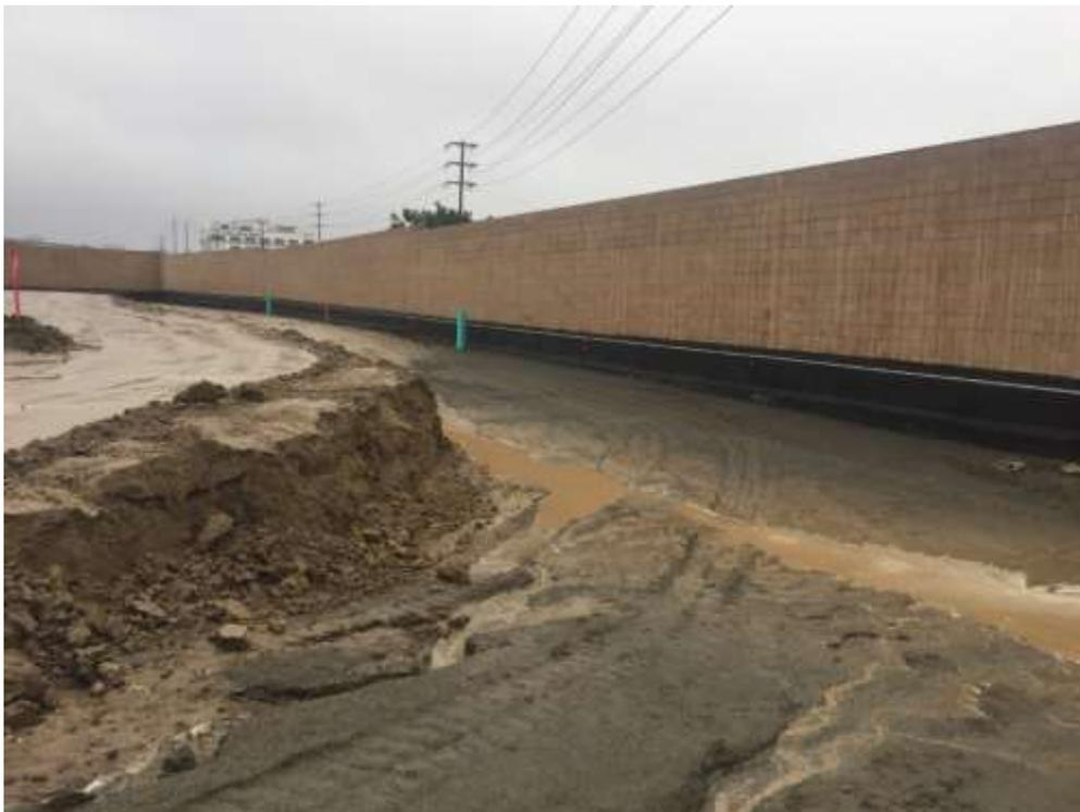
Figure 2 – Storm water drained into the lower corner of the site and into the drain system.
