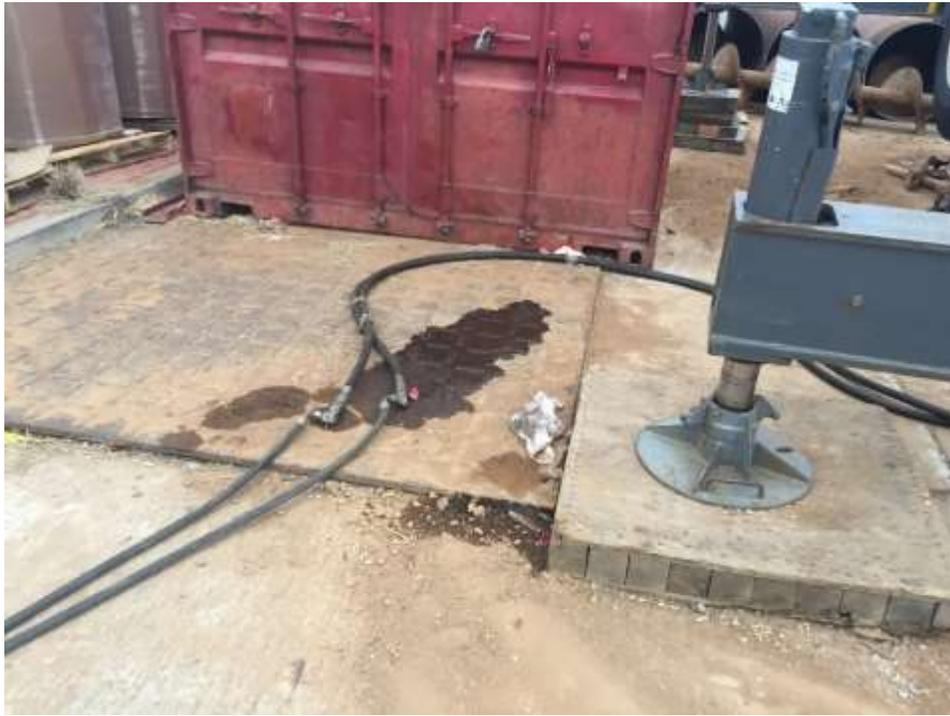
Figure 5 – Leaking hydraulic hoses at the jack and bore site with no spill containment as observed on May 17.
