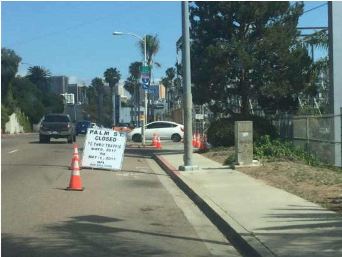
Figure 3 – Street closure signage in place for the jack and bore work. One lane of traffic is closed 24 hours a day during construction.
