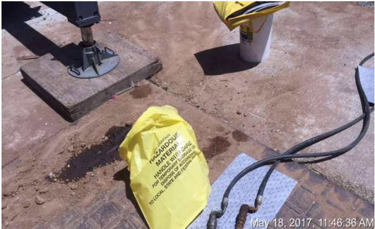
Figure 7 – Proper clean-up of the hydraulic leak was documented by SDG&E’s Environmental Inspectors on May 18 (photo courtesy of SDG&E).
