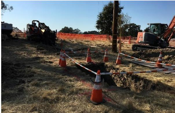
Figure 18. Horizontal Directional Drilling in field west of Substation, view west, October 31, 2017
