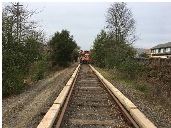
*Figure 23. Laying down planks along railroad tracks for crane to drive over, view north, December 19, 2017*
