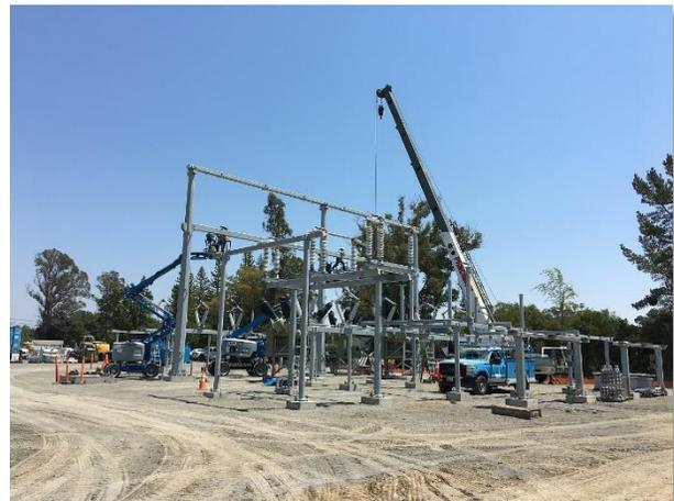
Figure 16. Erecting steel structures, installing insulators and switches, view southeast, August 1, 2017
