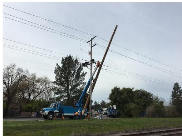
Figure 24. Replacing pole along Fulton No. 1 line, view west, January 29, 2018
