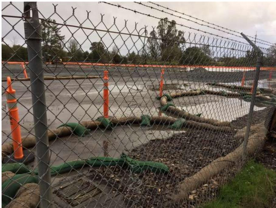
Figure 2 – Drainage inlets protected with BMPs on north side of substation site – view southwest, February 3, 2017.
