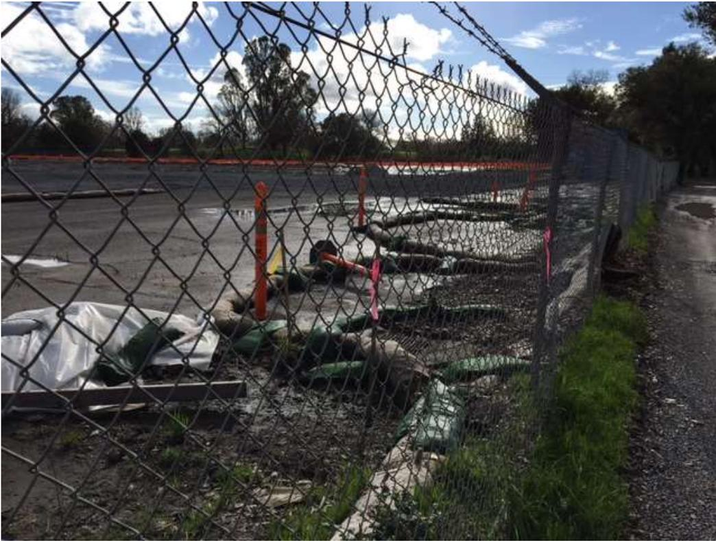
Figure 3 – Drainage inlets protected at substation site – view southwest, February 10, 2017.
