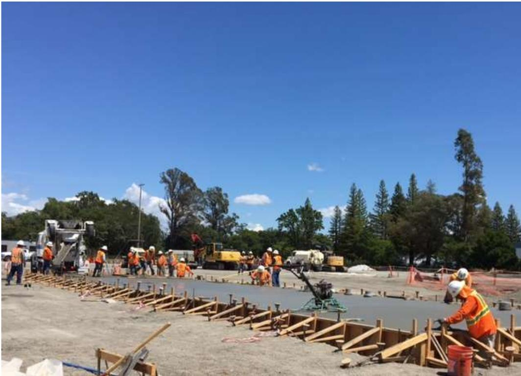
Figure 3 – Pouring and setting cement for switchgear foundation at substation site – view southeast, May 15, 2017.
