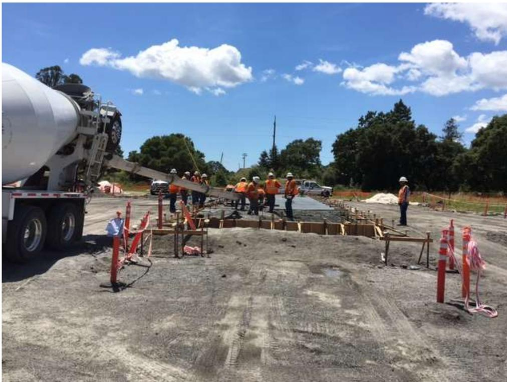
Figure 2 – Pouring cement for switchgear foundation at the substation site – view west, May 15, 2017.
