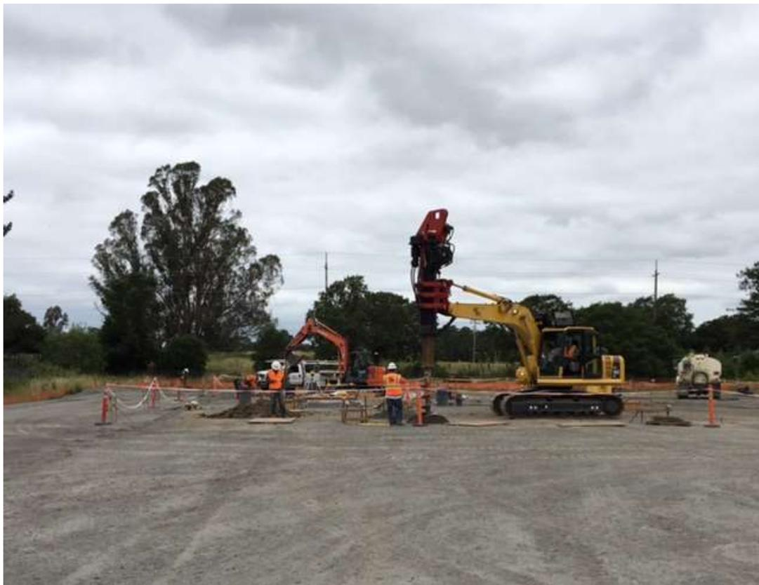
Figure 2 – Drilling pier holes on south side of substation site – view west, May 26, 2017.
