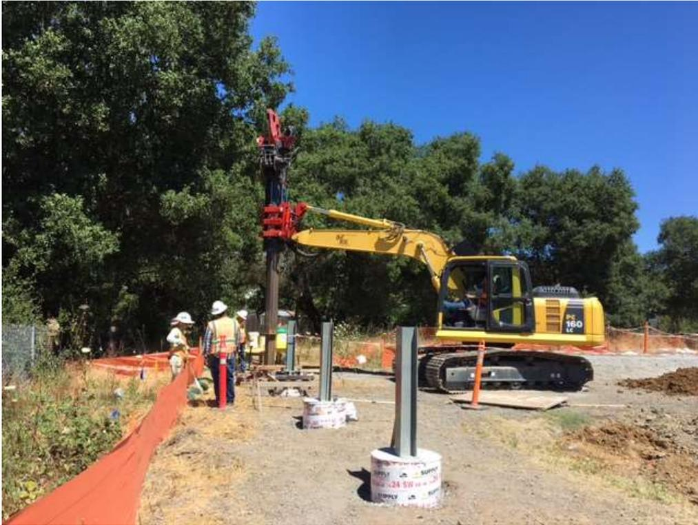
Figure 1 – Drilling foundation holes for perimeter wall piers in northwest corner of substation – view north, July 6, 2017.
