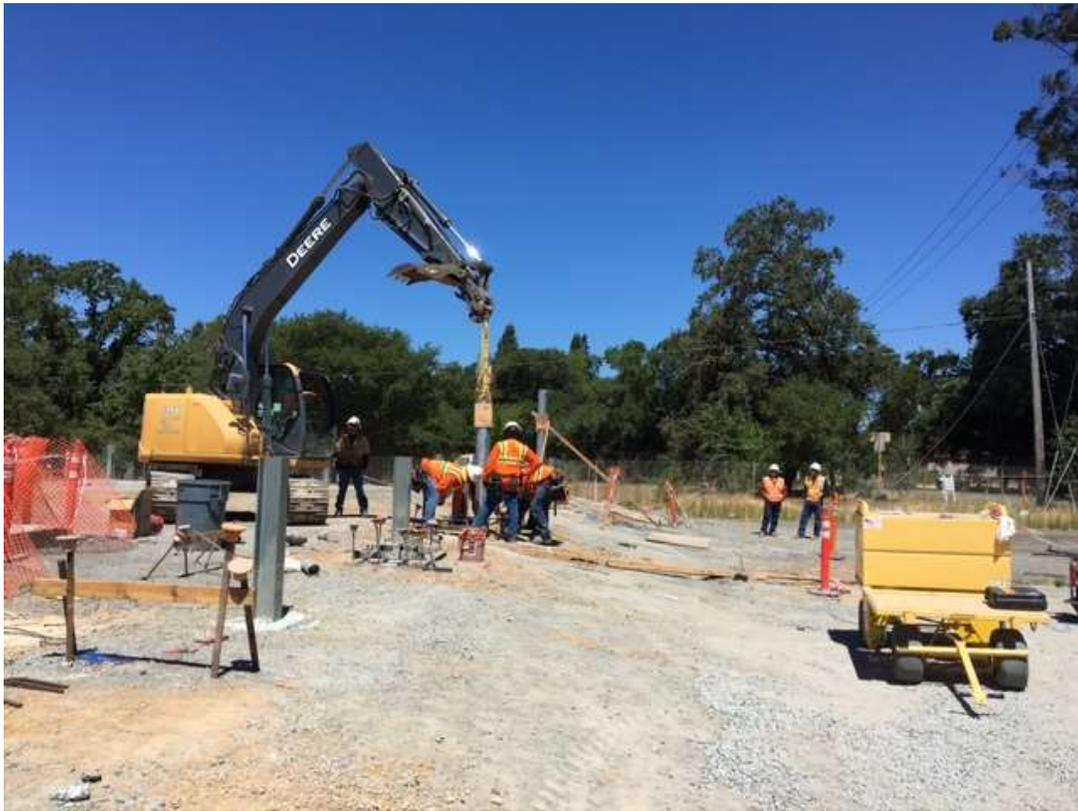
Figure 3 – Drilling pier holes for perimeter wall foundations on east side of site – view north, July 21, 2017.
