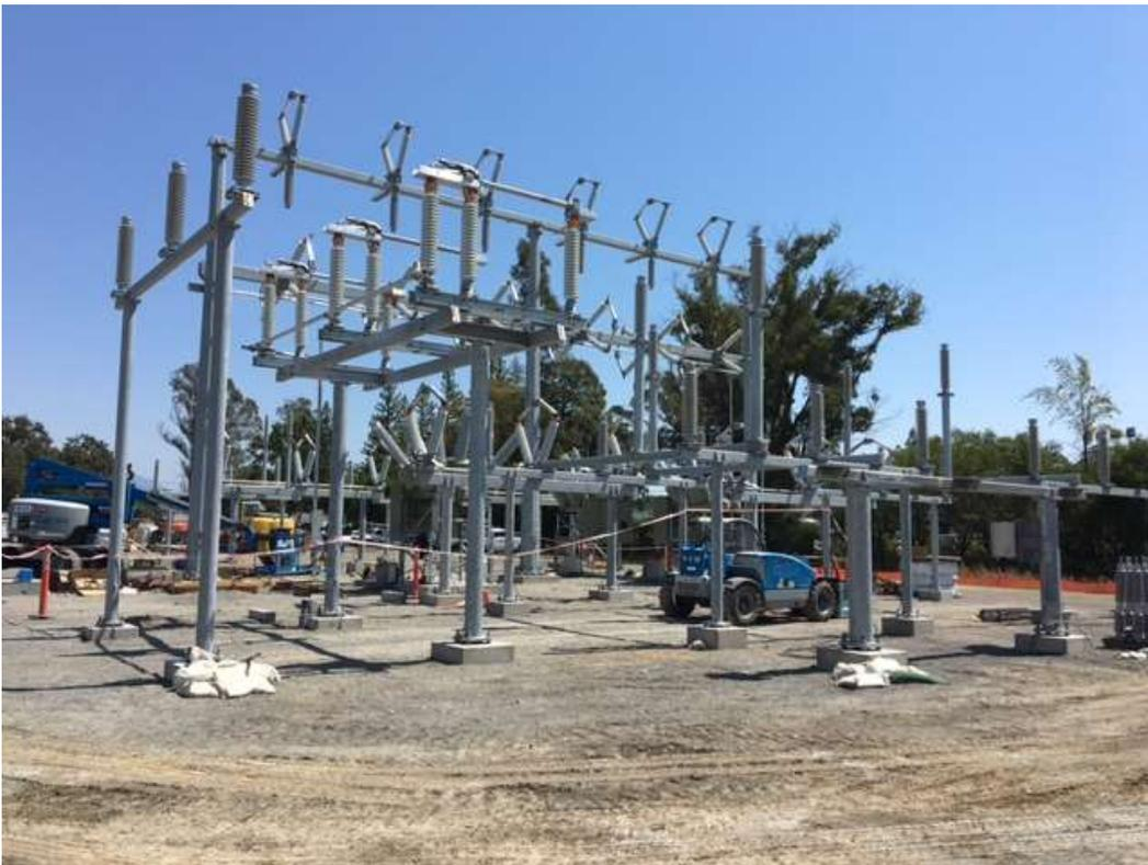
Figure 4 – Installation of switches and insulators on dead-end structures – view southeast, August 18, 2017.
