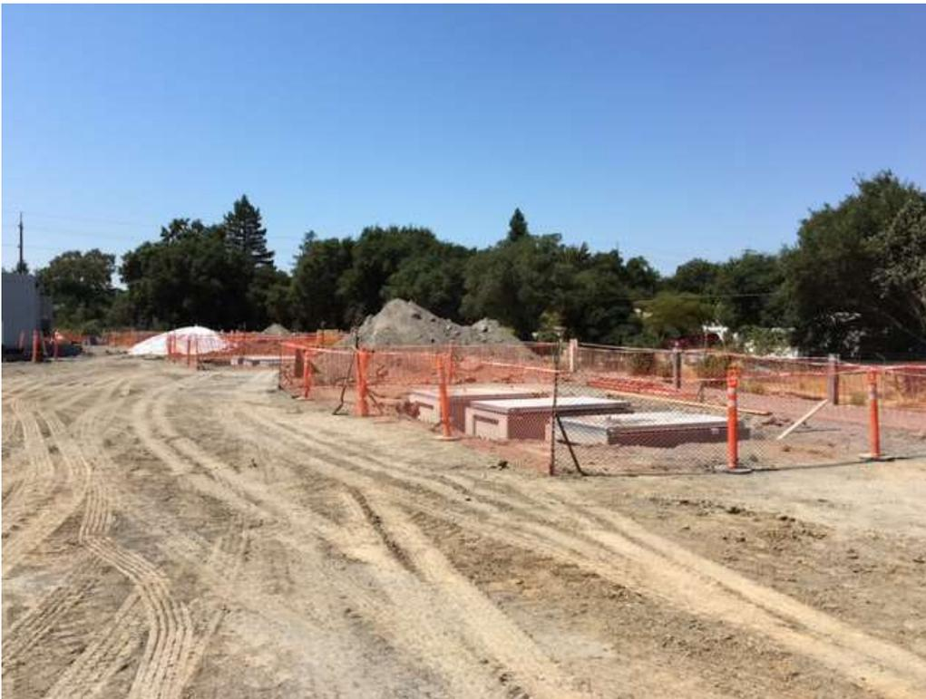
Figure 2 – Pull boxes set on northern perimeter – view northwest, August 18, 2017.
