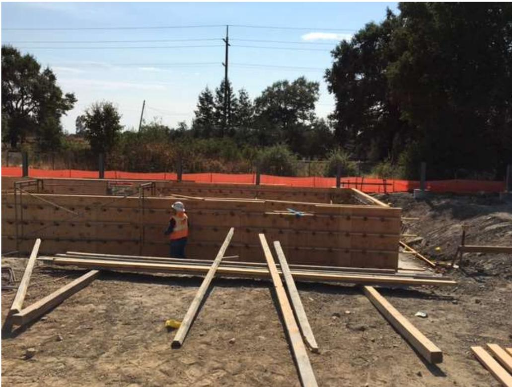
Figure 2 – Installing rebar and wall panel forms in the SPCC ponds – view west, September 6, 2017.
