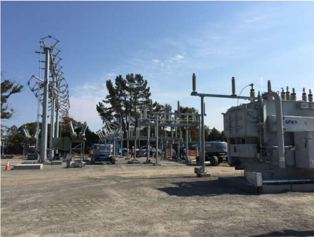
Figure 3 – Installing switches and insulators on dead-end structures – view south, September 6, 2017.
