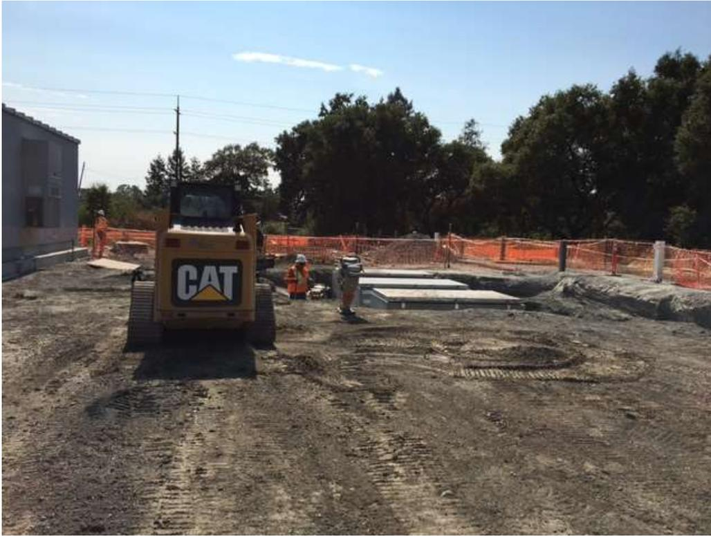
Figure 1 – Excavating trenches and installing conduit to pull boxes – view west, September 6, 2017.
