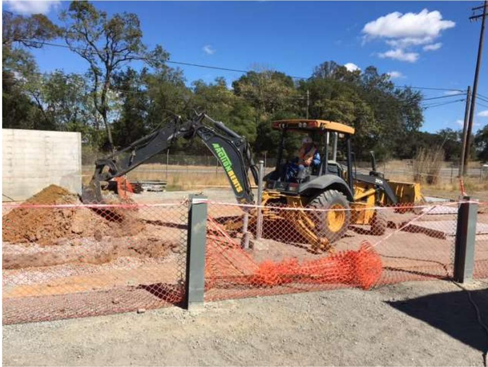
Figure 1 – Excavating conduit trenches and pull boxes – view east, September 21, 2017.
