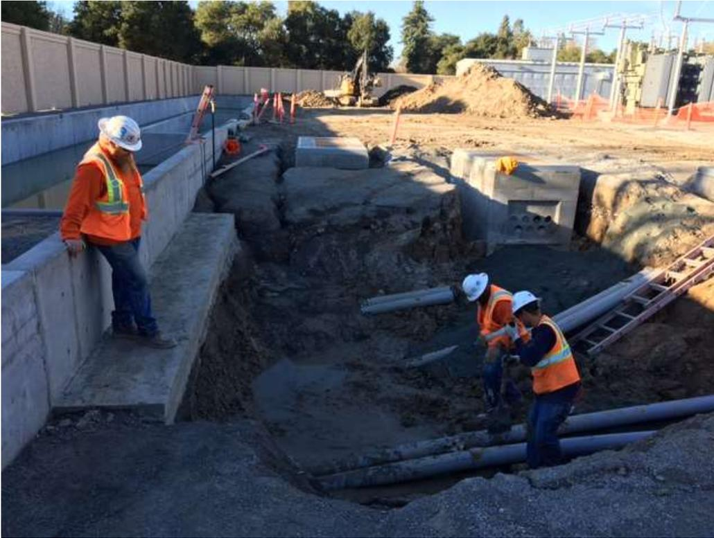
Figure 1 – Conduit installation to the pull boxes on the east side of the SPCC pond – view north, December 6, 2017.
