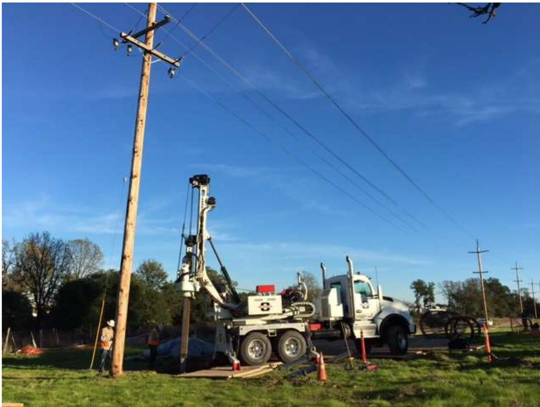
Figure 4 – Drilling for TSP in field west of substation site - view southeast, December 6, 2017.
