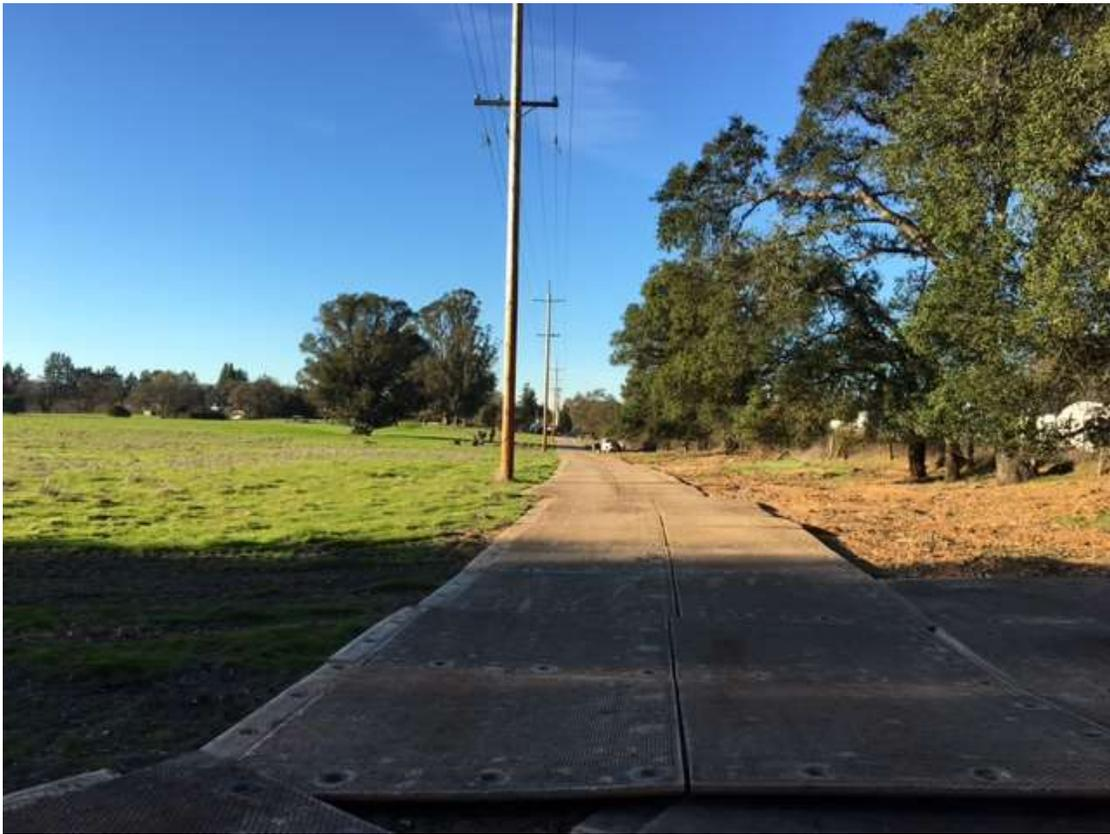
Figure 5 – Matting for equipment and vehicles to drive on to TSP location in field west of substation site - view north, December 6, 2017.
