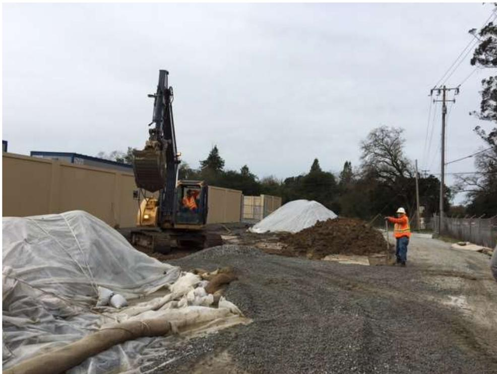
Figure 2 – Installing gravel outside Substation wall on east side – view north, January 29, 2018.
