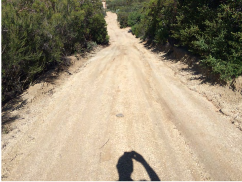
TL629E-06 - 60 feet west of Pole Z44177 looking west, minor rilling along north side of road
