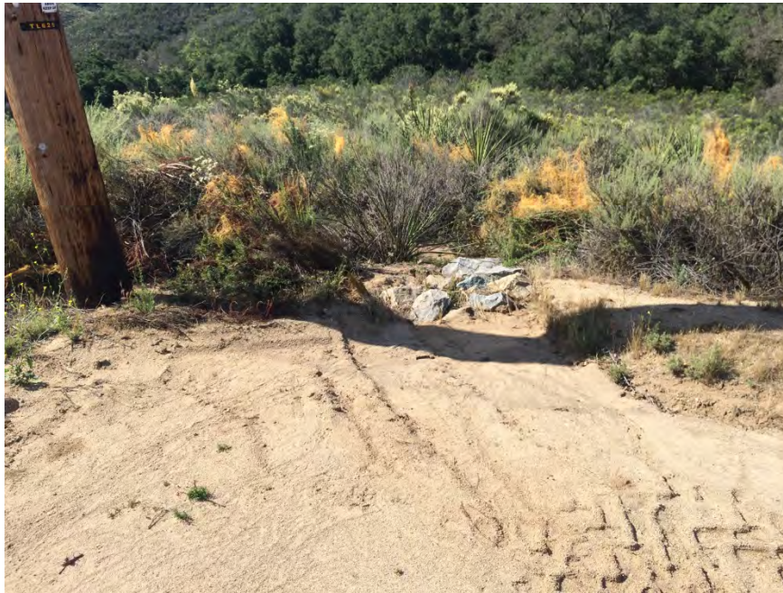
TL625B-09b – Riprap at outlet from pad at Pole Z272854
