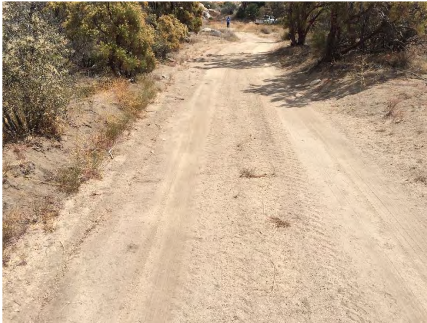
TL6931-09a - Along access road 390 feet south of tie-line between Pole Z44276 and Z44277, looking east, road in good condition with very minor rill on north side
