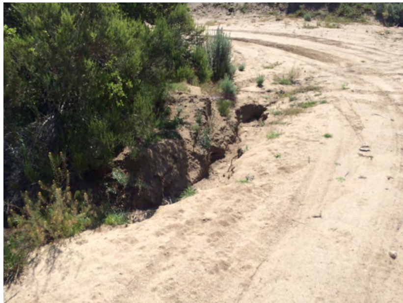
TL629E-11c – Incised area near intersection with dirt road 75' south of Pole Z442189, riprap to be added to incised area
