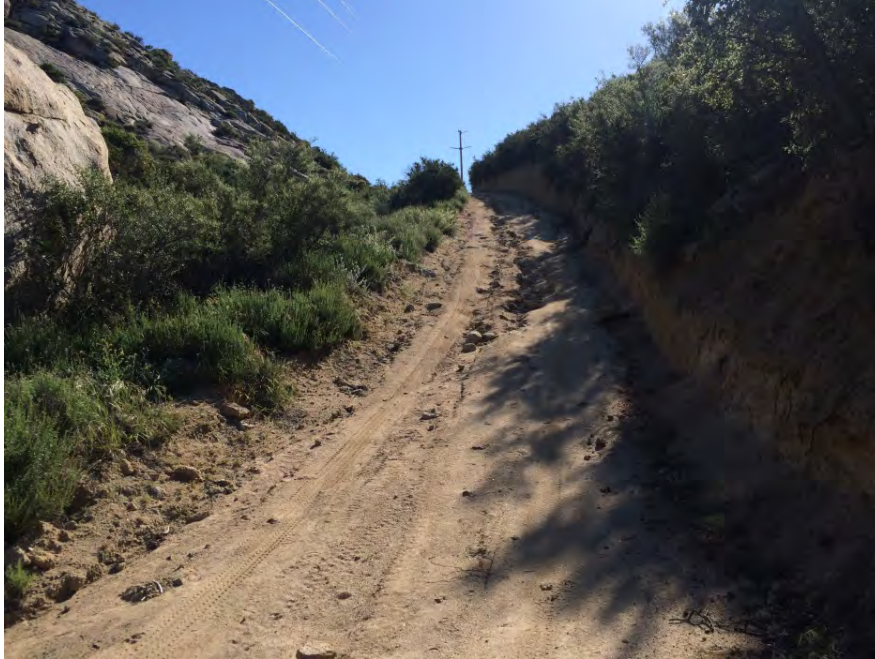
TL629E-03b - 300 feet east of Pole Z44165 looking east, rilling to be repaired and waterbar added during construction
