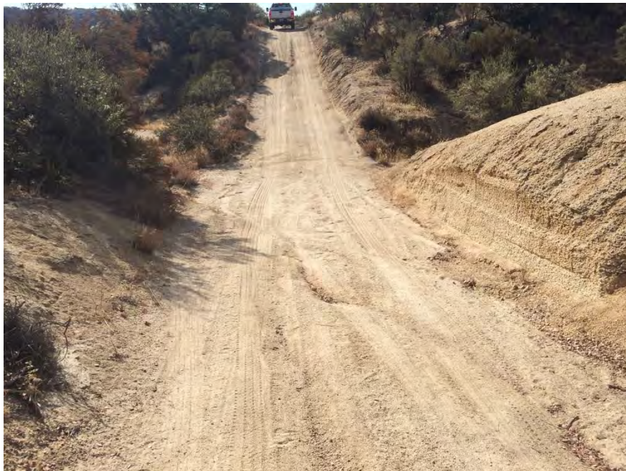
TL6931-01a – 60 feet southeast of Pole Z44241, looking southeast. Recommend adding rock at outlet of waterbar to capture runoff
