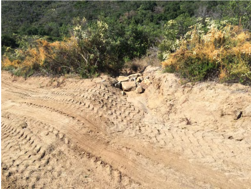
TL625B-10d - 115 feet north of Pole Z272855, waterbar outlet in good condition
