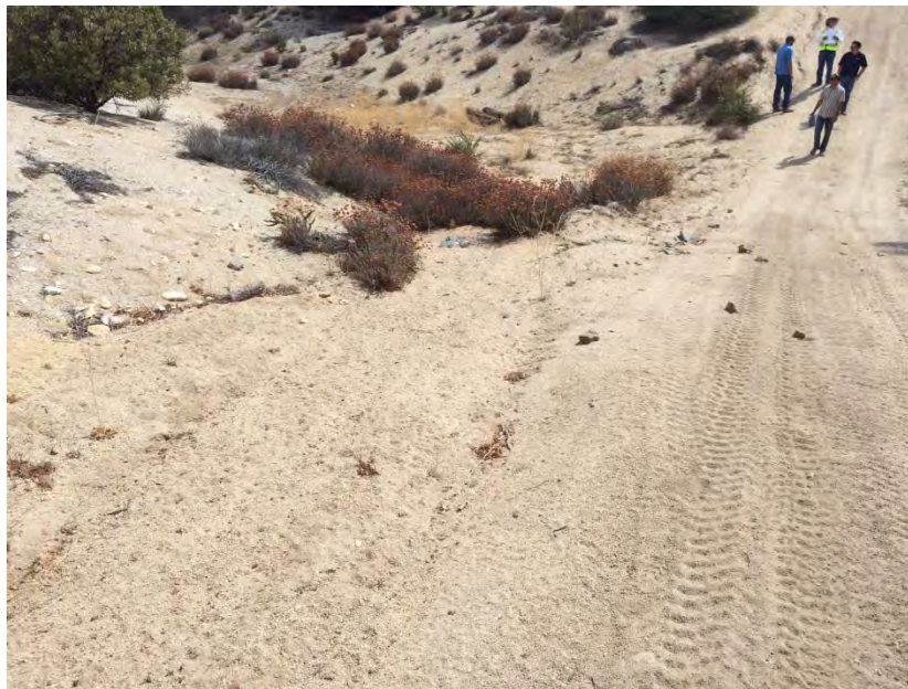
TL6931-07b - 140 feet east of Pole Z44272 looking east, sediment accumulation on north side of road at riprap noted and in need of cleanup
