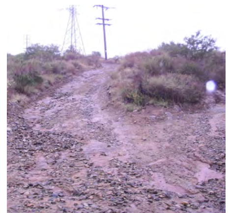
Example of maintenance road primarily composed of rock and gravel.
