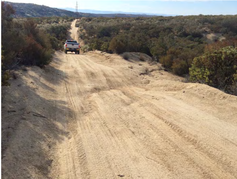
TL6931-01a – 60 feet southeast of Pole Z44241, looking southeast. Recommend adding rock at outlet of waterbar to capture runoff
