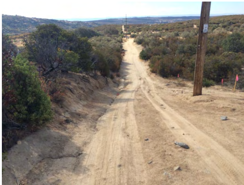
TL6931-03a – Near Pole Z44244 looking southeast, waterbar at top of hill upstream of evaluated area in good condition
