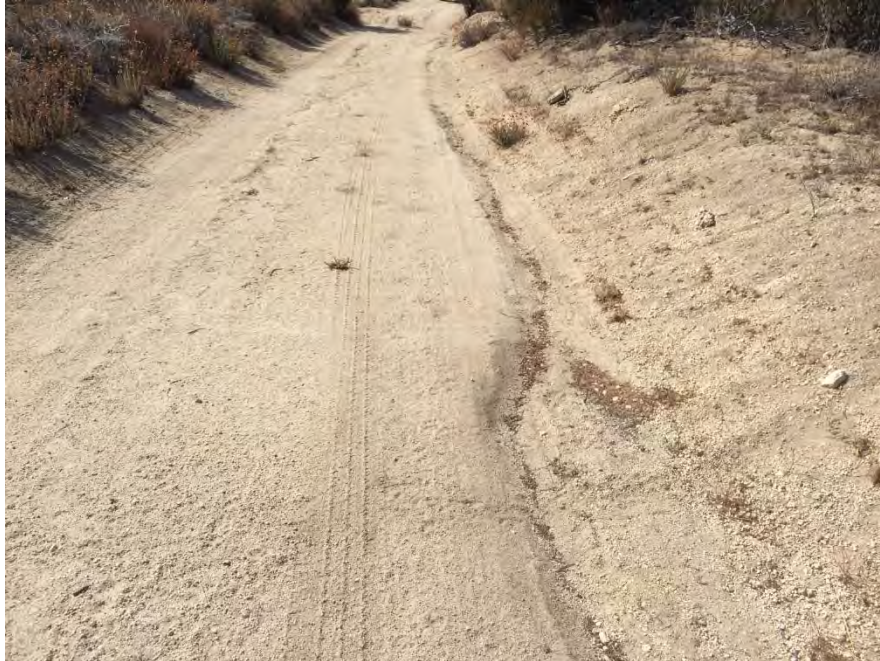
TL6931-05a – 120 feet south of Pole Z44248 looking south, minor rilling noted
