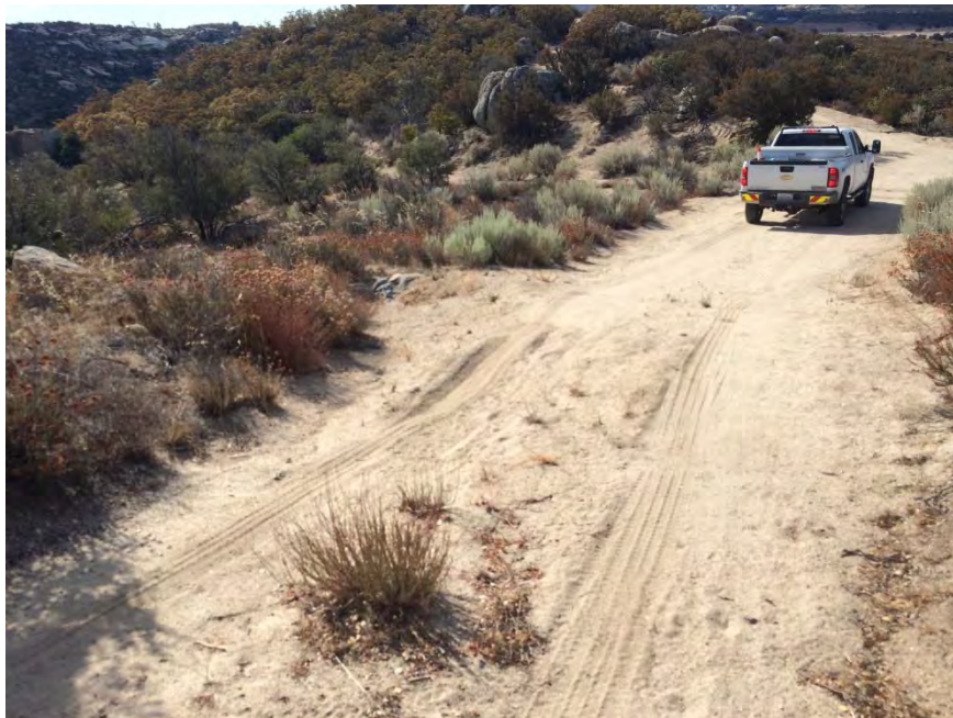
TL6931-05a – 120 feet south of Pole Z44248 looking south, minor rilling noted
