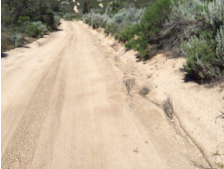
TL629E-09e - 200 feet east of Pole Z44184 looking west, minor rilling along north side of the road
