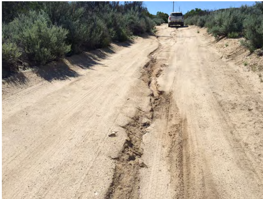
TL629E-10d - 140 feet north of Pole Z44187 looking south, runoff causing rilling across the road. Would be alleviated by improvement/repair to waterbar upstream
