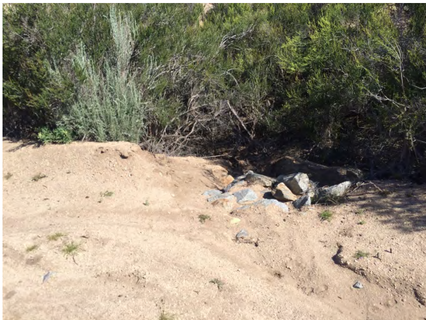
TL629E-07c - 100 feet west of Pole Z44178-79, sediment accumulation in riprap to be cleaned out
