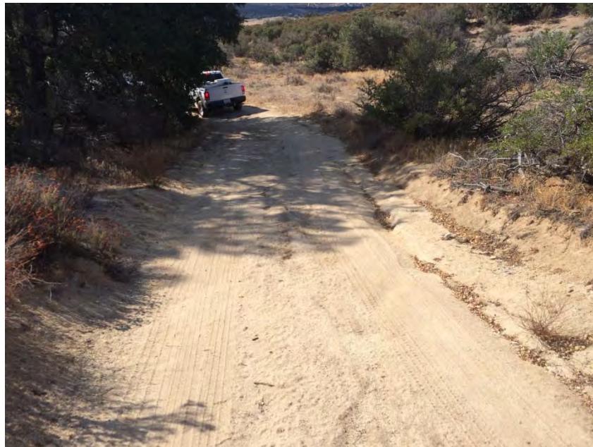
TL6931-04a – Along access road 900' west of tie-line/Pole Z44248, 160' south of road intersection, looking south, minor rilling noted
