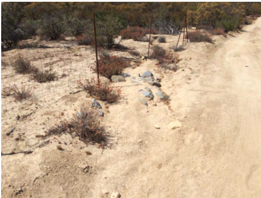
TL6931-11c - 65 feet west of Pole Z44281, sediment accumulation in waterbar on south side of the road, recommend cleaning out
