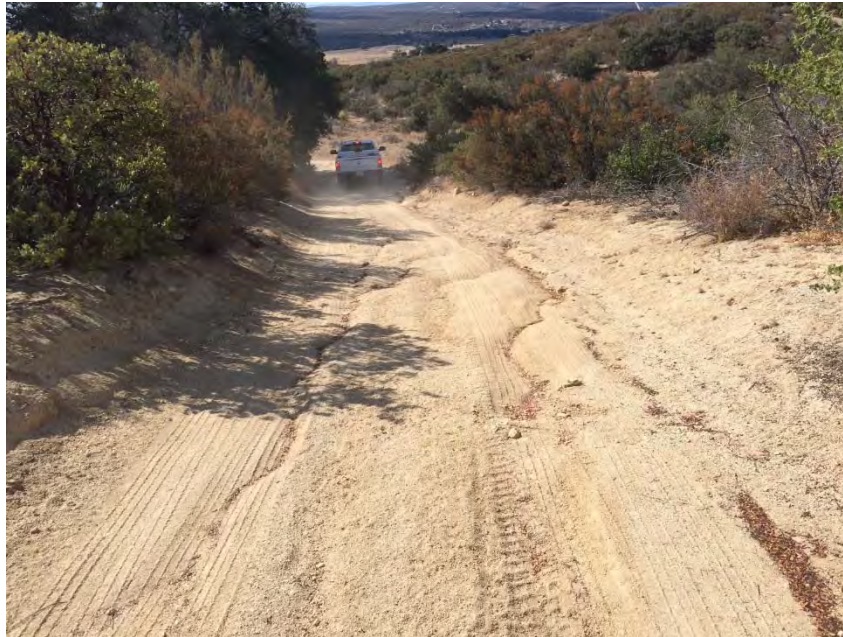
TL6931-04a – Along access road 900' west of tie-line/Pole Z44248, 160' south of road intersection, looking south, minor rilling noted
