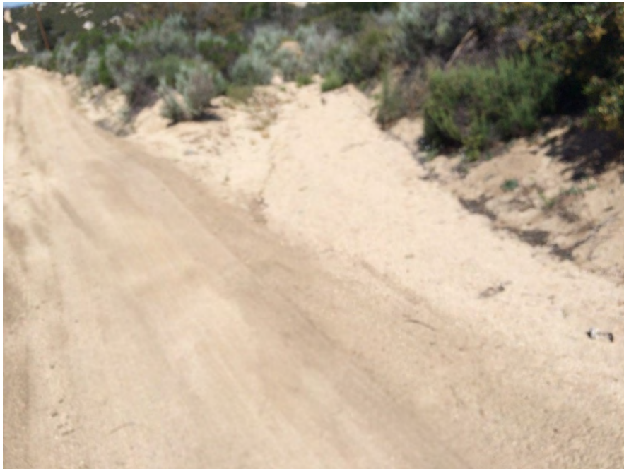
TL629E-09e - 200 feet east of Pole Z44184 looking west, minor rilling along north side of the road
