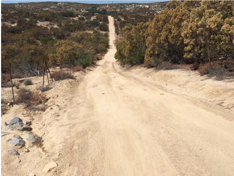
TL6931-11b - 65 feet west of Pole Z44281 looking west, minor rill along north side of road
