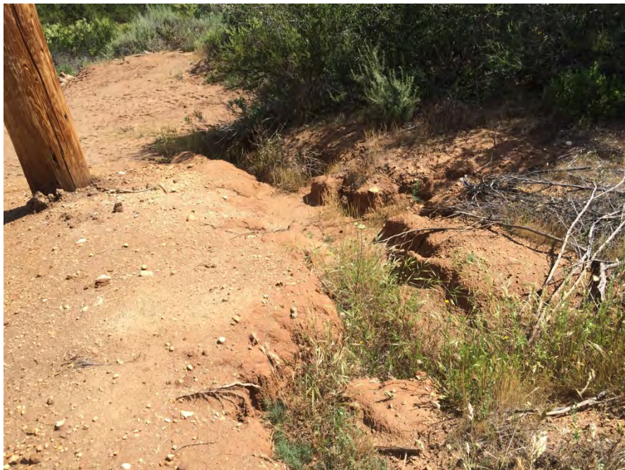
TL625B-15e – Midway between Poles Z272866 and Z272867, rilling noted near existing pole slated for removal. Pad area to be restored through Habitat Restoration Plan
