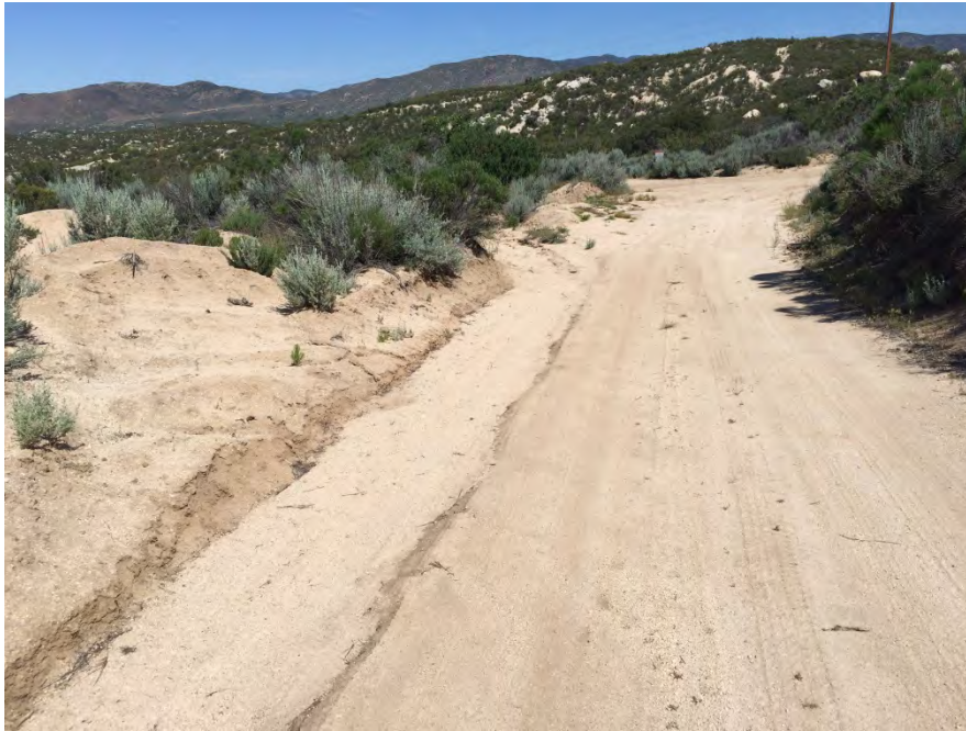
TL629E-10a - 130 feet south of intersection with non-SDG&E dirt road looking north, sediment accumulation within rilled area at west side of road. Sediment to be cleaned out, velocity check dams to be added
