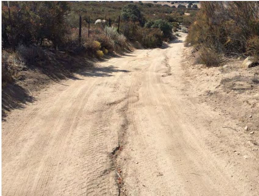
TL6931-06a – Along access road 130' west of tie-line, opposite midpoint between Poles Z44252 and Z44253, looking south, minor rilling noted
