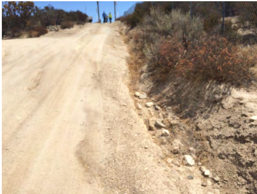
TL6931-13a - 210 feet west of Pole Z44284_85 looking east, road in good condition with minor rill along south side
