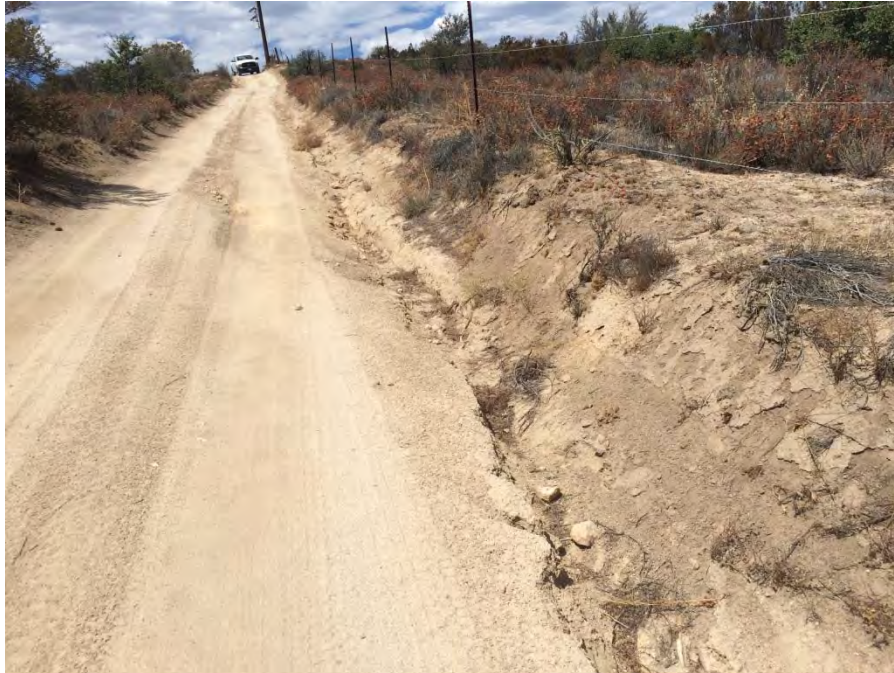
TL6931-12c - 290 feet east of Pole Z44281 looking west, road in good condition with minor rill along north side
