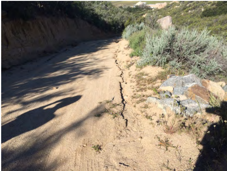
TL629E-03c - 490 feet east of Pole Z44165 looking east, waterbar to be lowered to allow runoff to exit the roadway
