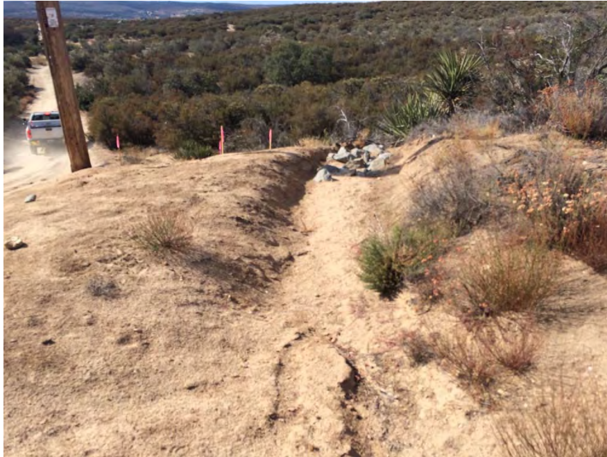
TL6931-03a – Near Pole Z44244 looking southeast, waterbar at top of hill upstream of evaluated area in good condition
