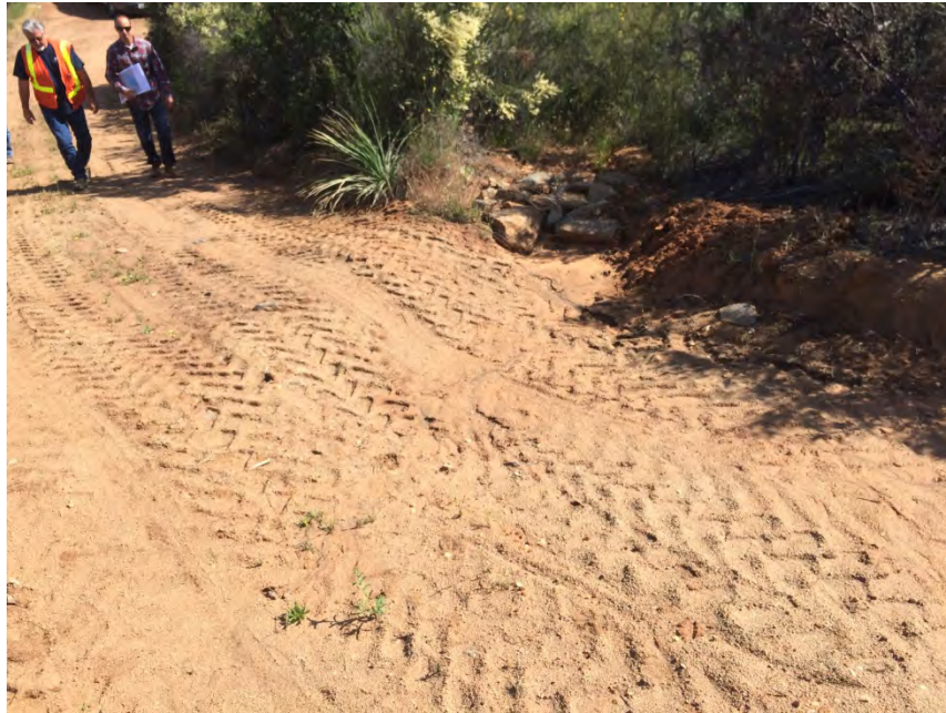
TL625B-07b - 300 feet north of Pole Z272854, typical waterbar in good condition
