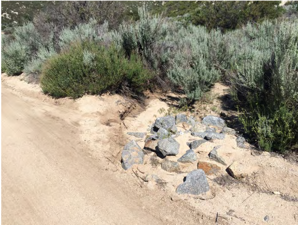
TL629E-09c – 60 feet west of Pole Z44184, rilling at outlet from riprap
