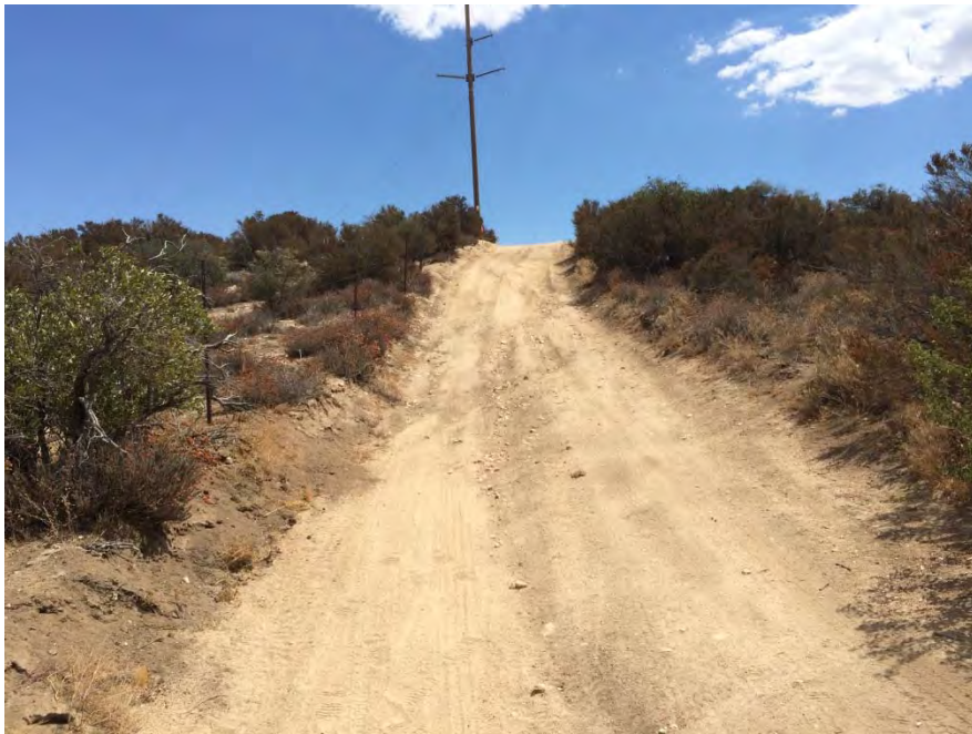
TL6931-10b – 150 feet west of Pole Z44284_85 looking east minor rill noted in center of road
