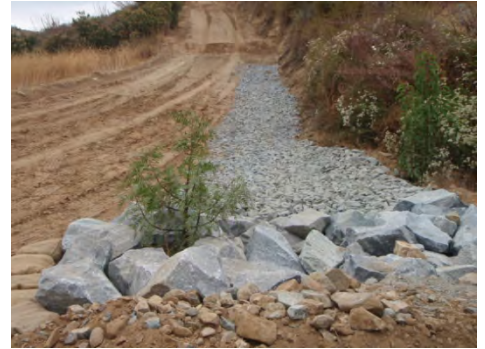
Example of a rip rap (or stabilized) drainage swale.
