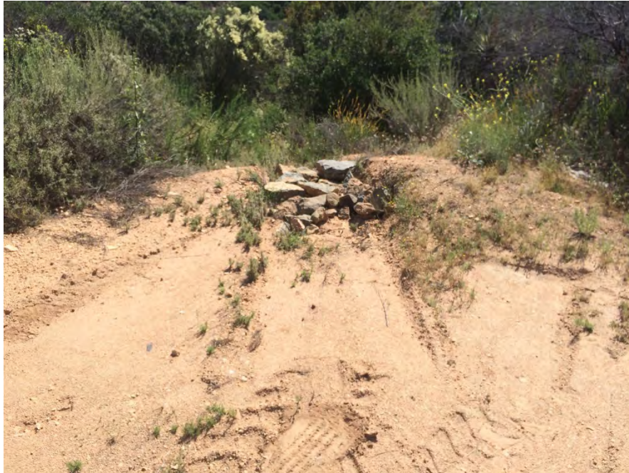
TL625B-06b – Riprap at outlet from pad at Pole Z272853
