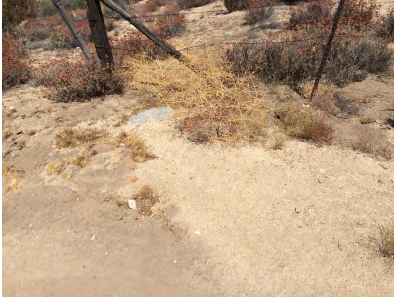
TL6931-10c – 35 feet east of Pole Z44282_83 looking west, sediment accumulation downstream of evaluated road reach, recommendation to clean out of waterbar
