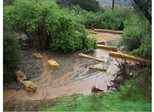
Example of rice hay bales effectively reducing runoff velocity and settling out debris and sediment.
