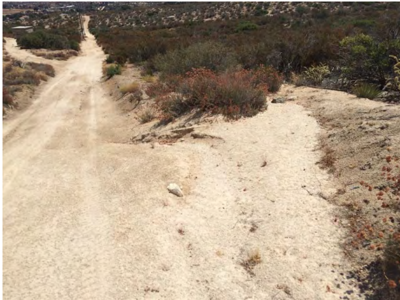
TL6931-14c – 140' east of Pole Z44284_85 looking east, sediment accumulation in waterbar and recommend cleaning out
