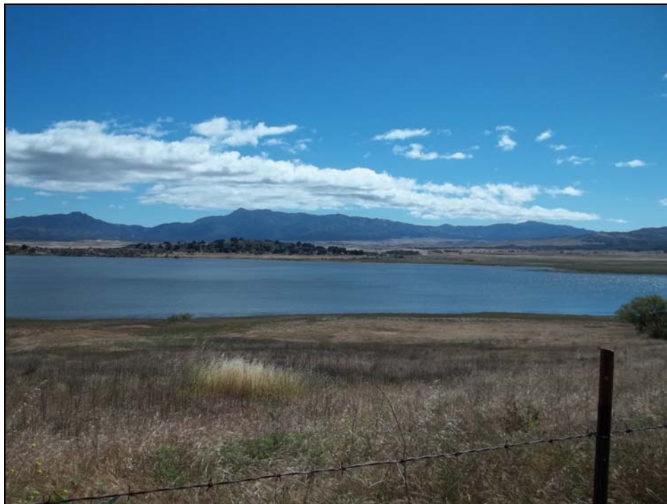
Photograph 4. View of TL-682 traversing Lake Henshaw.
