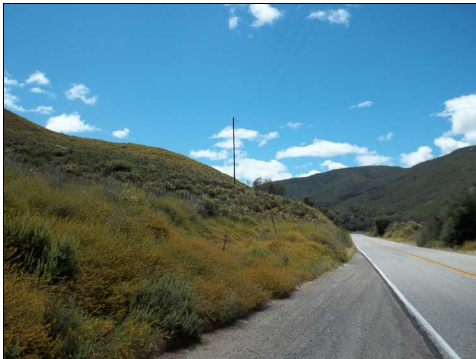
Photograph 2. View of TL-628 looking east in the La Jolla Indian Reservation.
