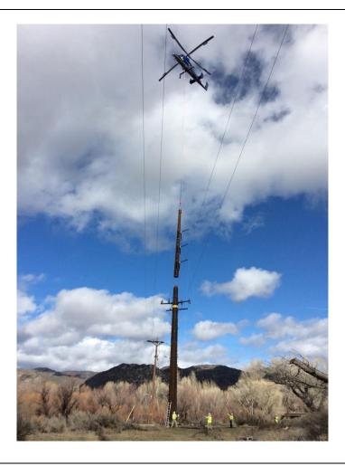
**Photo 2:** A construction crew observed utilizing helicopter external load operations to set a new steel pole at Pole Z100056 (TL 629C).
