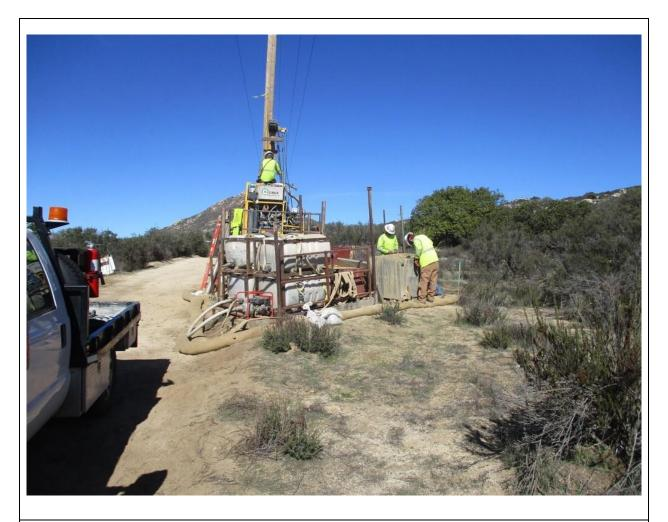
**Photo 5:** During micropile foundation hole drilling at Pole Z41007, the construction crew was observed cleaning out the cuttings containment box, which is used to trap drill cuttings and control dust emissions in accordance with APM AIR-05.
