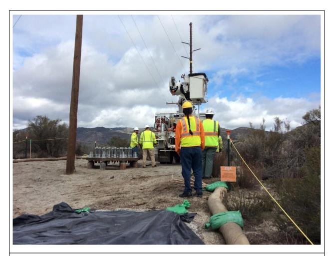
**Photo 1:** A construction crew observed setting up a bucket truck in order to spread wire at Pole Z100051 (TL 629C). Archeological and Native American monitors were on-site monitoring the activity, and ensuring that no disturbance occurred to an adjacent cultural ESA in accordance with the HPMP, MM CUL-1, and APM CUL-04.
