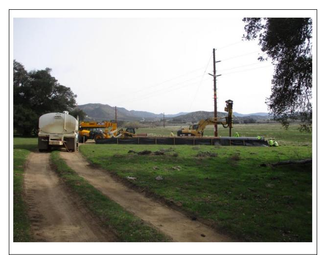
**Photo 5:** Construction crews were observed drilling for a direct bury pole hole at Z409970. Silt fence was observed in good condition in accordance with the SWPPP.
