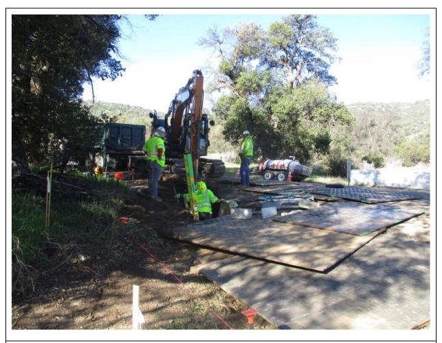
**Photo 1:** Construction crews were observed trenching for the installation of 12 kV underground line at C449. Due to the presence of a cultural resources ESA within 50 feet, an archeological and Native American monitor were observed inspecting excavated soils in accordance with the HPMP, MM CUL-1, and APM CUL-04.
