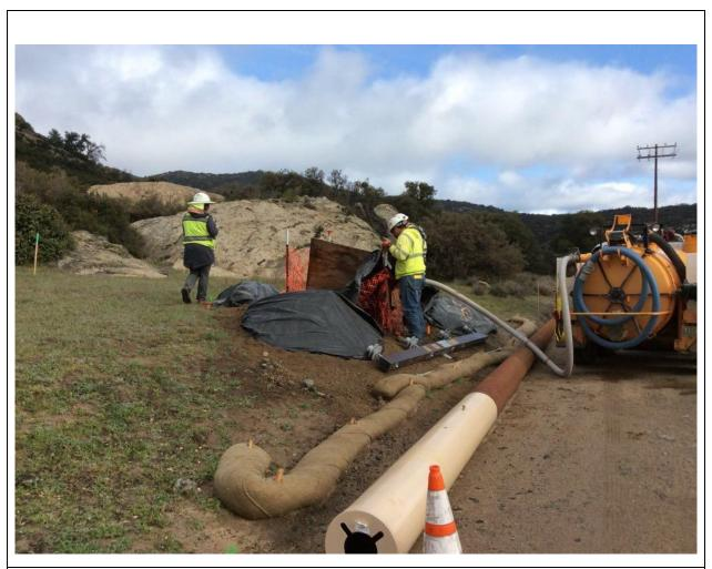
**Photo 3:** A construction crew was observed pumping groundwater out of the pole excavation at P258869 (C 449) prior to pole setting. A Biological Monitor was present in accordance with MM BIO-22 and the spoils stockpile was observed to be securely covered in accordance with the Erosion Control Plan and SWPPP. The water was transported in the vacuum machine to Buckman Springs Fly Yard, where it was dispersed for dust control in accordance with APM AIR-02.
