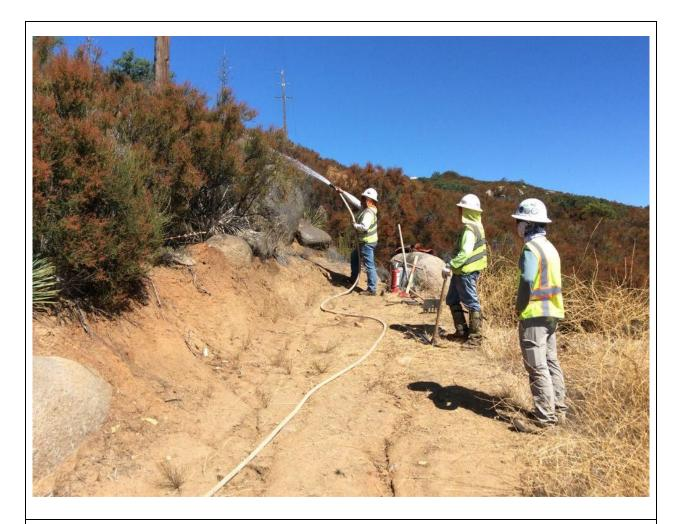
**Photo 4:** In preparation for vegetation clearing and chipping at Pole Z272992 (TL 625C), the area was wet down in accordance with the CFPPP Fire Matrix (MM FF-1) for chipping work on private land with a FPI of Elevated.
