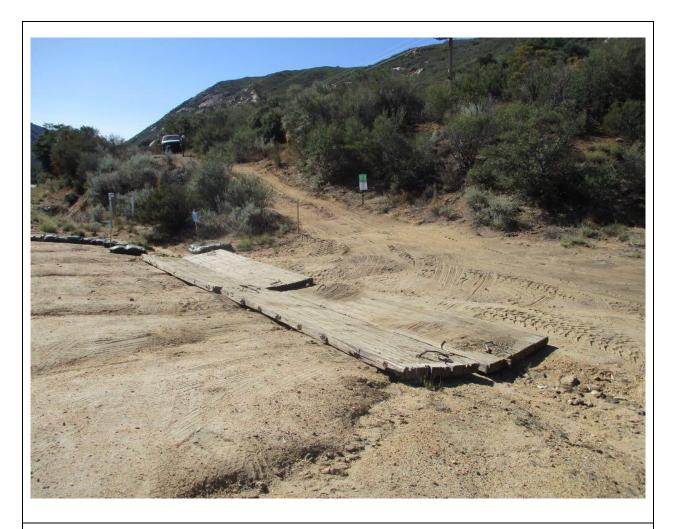
**Photo 5:** During micropile drilling at Pole Z40255 (TL 629A), a jurisdictional drainage crossing along the site access road was flagged, gravel bags were installed, and timber mats were used to prevent impacts to the stream channel in accordance with APM HYD-06.
