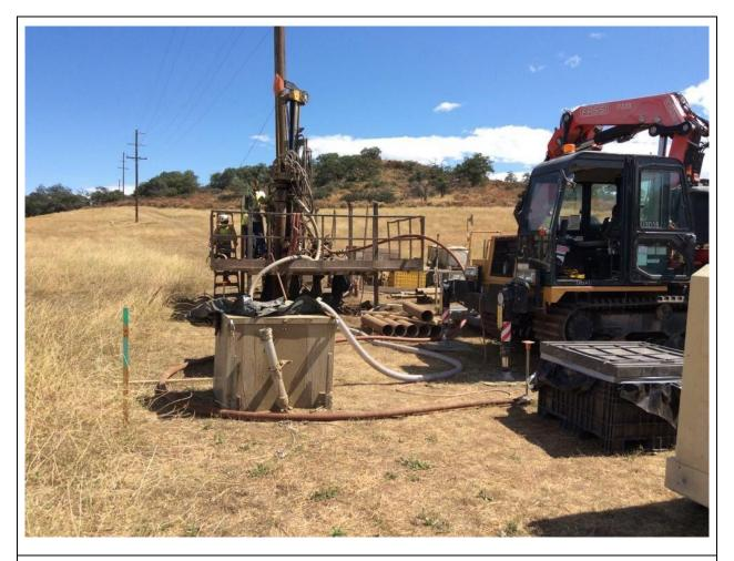
**Photo 1:** During drilling for a micropile foundation at Pole Z272950 (TL 625C), a crew was observed using a containment box to trap drill cuttings and reduce dust emissions from drilling in accordance with APM AIR-05.
