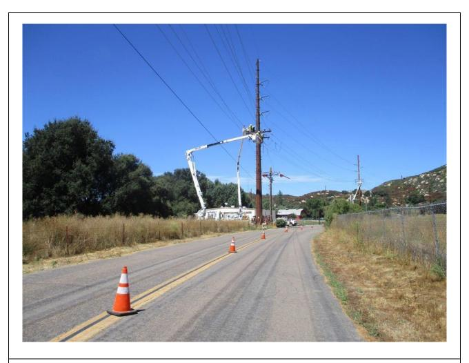
**Photo 6:** Construction crews observed dead-ending 12 kV lines at Pole Z872453 and Pole Z872452 (TL 629A). A Pro Traffic crew directed one-way traffic around staged equipment on River Drive in accordance with APM TRANS-02.
