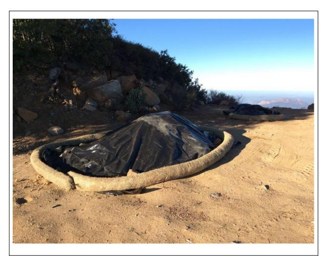
**Photo 5:** Dirt stockpiles staged within a stringing site on Lookout Road (C 79A) were covered with plastic sheeting and surrounded by fiber rolls in accordance with the Erosion Control Plan and Storm Water Pollution Prevention Plan (MM HYD-01, MM BIO-7), and APM HYD-09.
