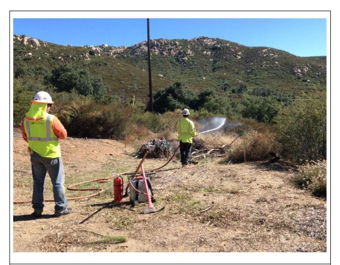
**Photo 4:** In preparation for vegetation clearing and chipping on the access road to Pole P119857 (TL 625C), the area was wet down in accordance with the CFPPP Fire Matrix (MM FF-1) for chipping work on private land with a FPI of Elevated.
