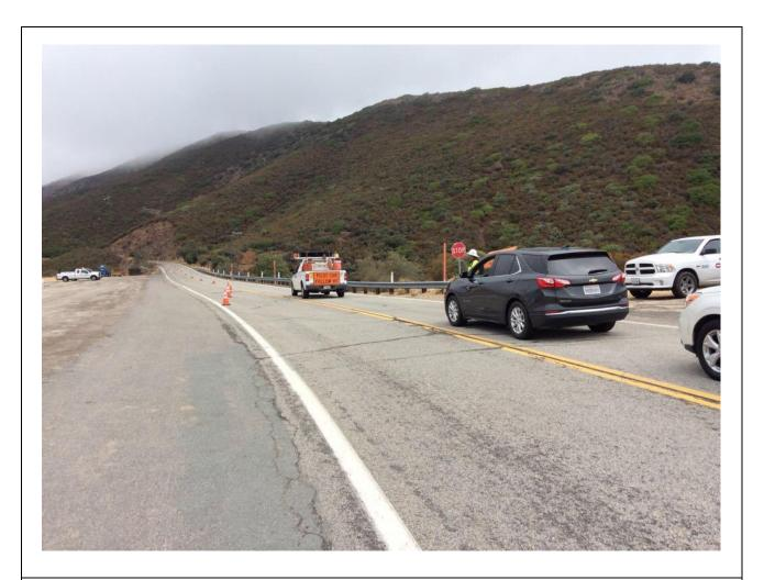
**Photo 6:** A clearly marked pilot vehicle was used to shuttle traffic through the construction zone along Sunrise Highway where one lane was closed for trenching activities (C 440) in accordance with the TCP (APM TRANS-05).
