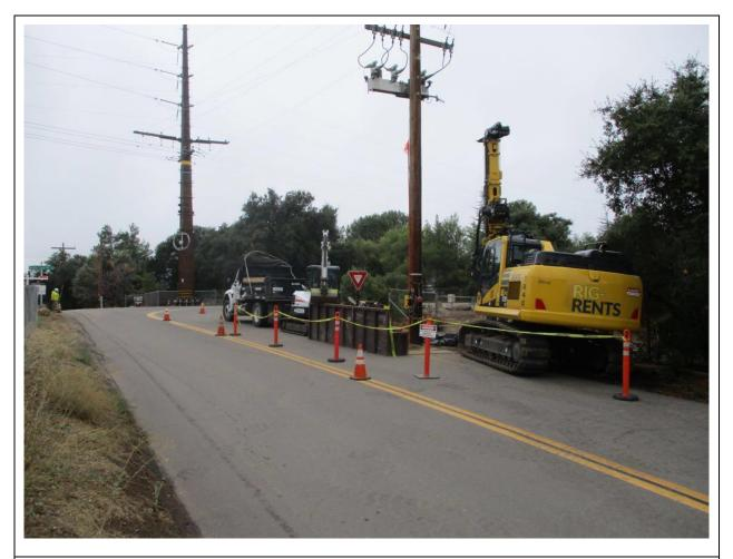
**Photo 1:** During direct bury pole hole drilling at Pole Z172738 (TL 629A), the crew was observed exporting spoils using a haul truck with a load cover in accordance with APM AIR-02.
