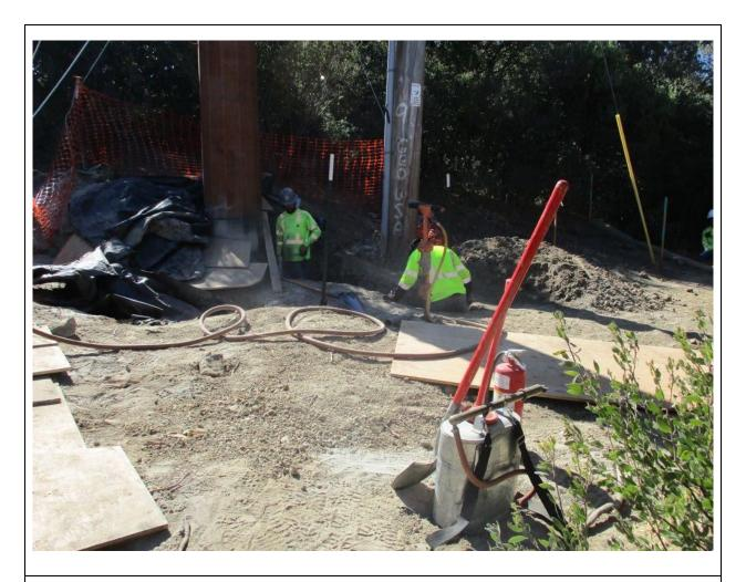
**Photo 4:** During intercept installation at Pole Z172741 (TL 629A), a set of fire tools was observed within 50 feet of the activity in accordance with APM HAZ-04 and the CFPPP (MM FF-1).
