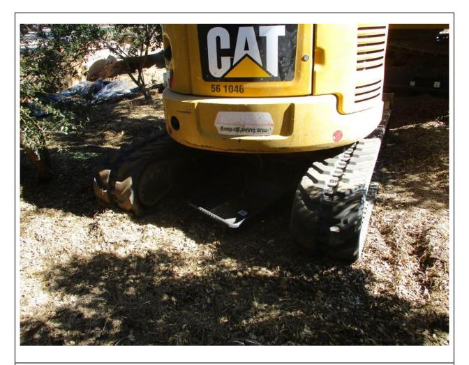
**Photo 5:** During pole hole drilling at Pole Z172739 (TL 629A), the crew was observed using a drip pan beneath staged equipment to prevent leaks or spills from being discharged into the soil in accordance with MM PHS-2.
