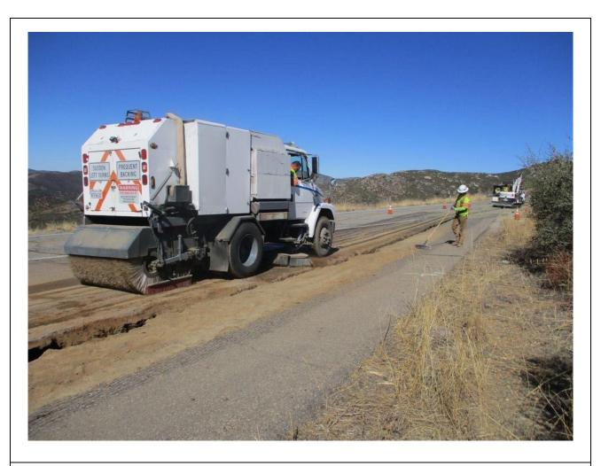
**Photo 6:** After trenching for the underground distribution line at C 440 (Phase 1), a street sweeper was observed being operated along Sunrise Highway to clean the road and prevent off-site erosion in accordance with the ECP (MM HYD-1) and SWPPP (MM BIO-7).
