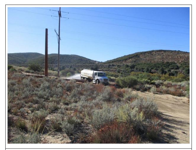
**Photo 1:** Prior to crew ingress into Pole Z276634 (TL 629A), a water truck was observed wetting down the area to prevent dust emissions in accordance with APM AIR-02 and APM AIR-05.
