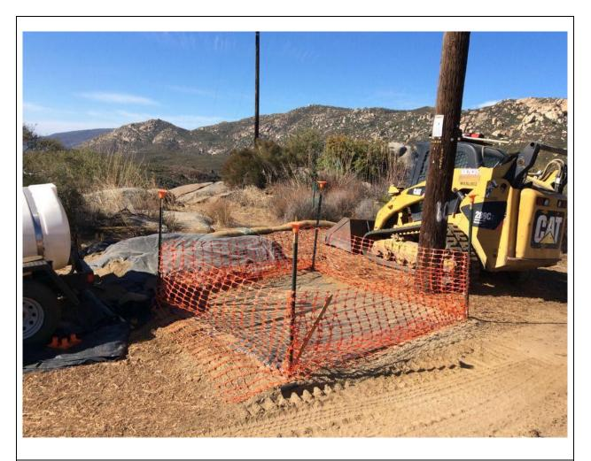
**Photo 2:** The pole hole at Pole Z273006 (TL 625C) was observed to be securely covered to prevent wildlife entrapment in accordance with MM BIO-23.
