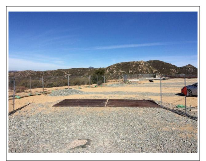
**Photo 5:** The entrance to Staging Yard 2A (C 440) was observed to be stabilized with rattle plates and rock aprons in accordance with project Erosion Control Plan (ECP), SWPPP (MM HYD-01, MM BIO-7), and APM HYD-09.
