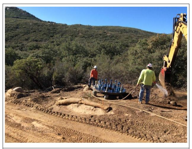
**Photo 1:** A crew at Pole Z293927 (TL 625C) was observed using water to minimize dust emissions during ground rod trenching in accordance with APM AIR-05.
