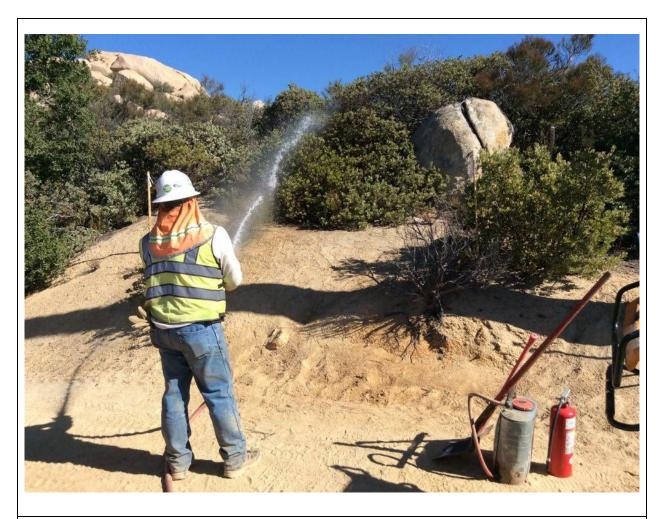
**Photo 4:** A crew member was observed wetting down vegetation prior to removal and chipping at Pole Z273018 (TL 625C) in accordance with the CFPPP Fire Prevention Matrix for the activity on NFS land with a Project Activity Level (PAL) D. In addition, a complete set of fire tools was observed on site.
